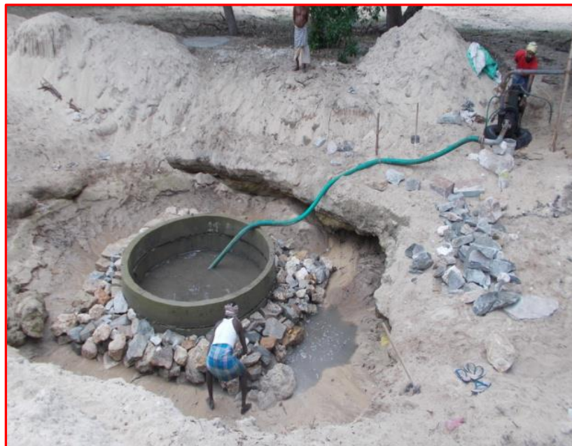
Siphoning out the water for construction of the Teertham
