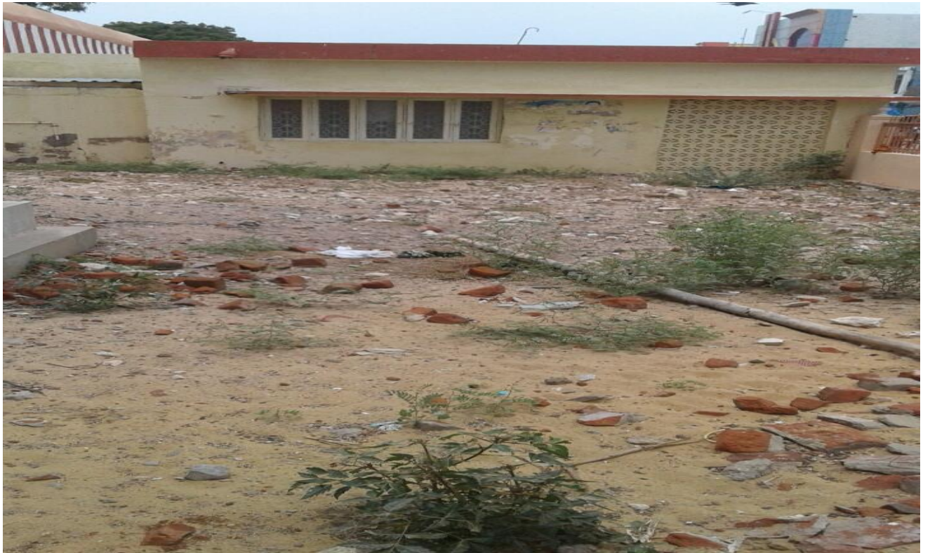
Another view of the South tower
