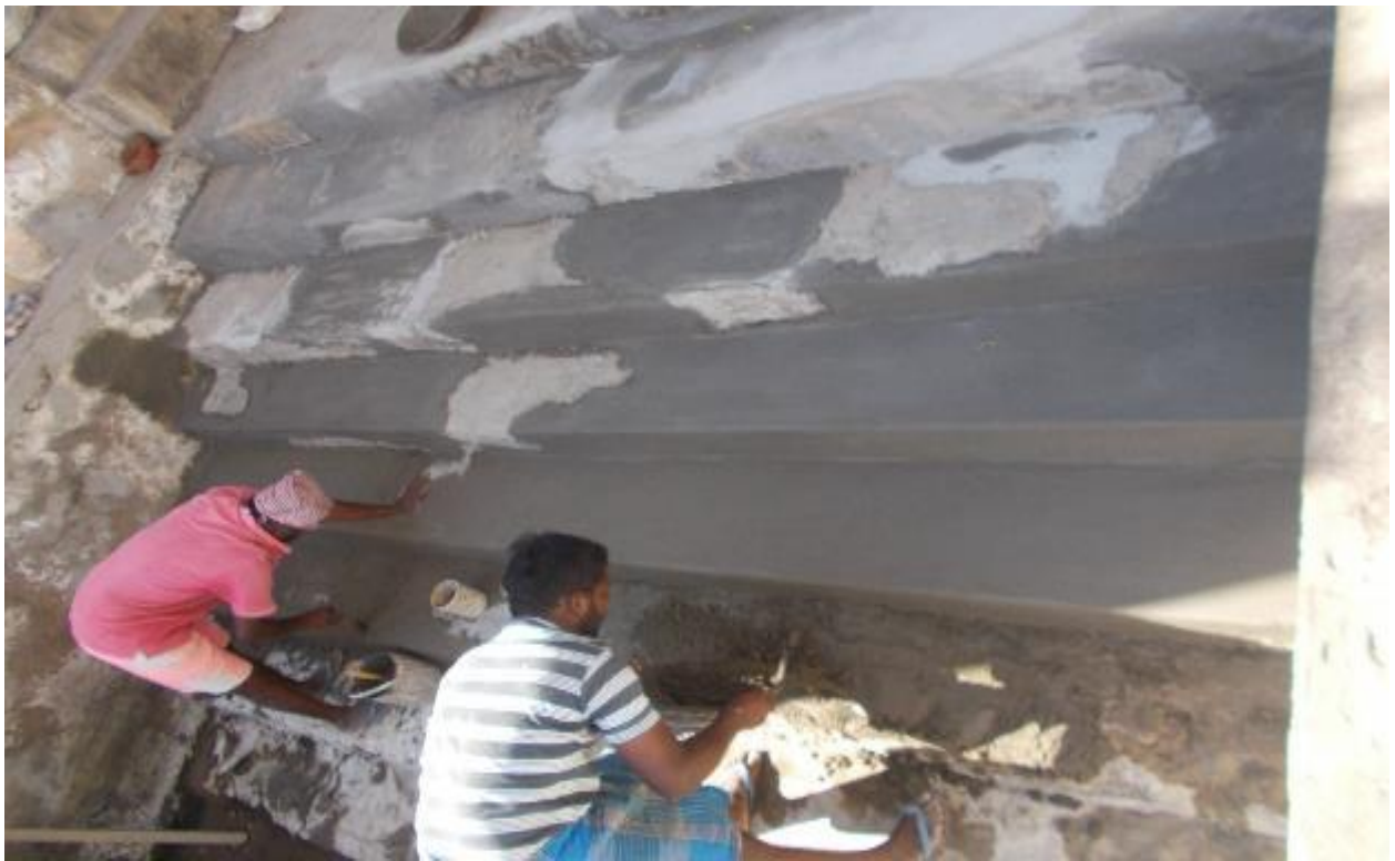
Repairing of Stairs
