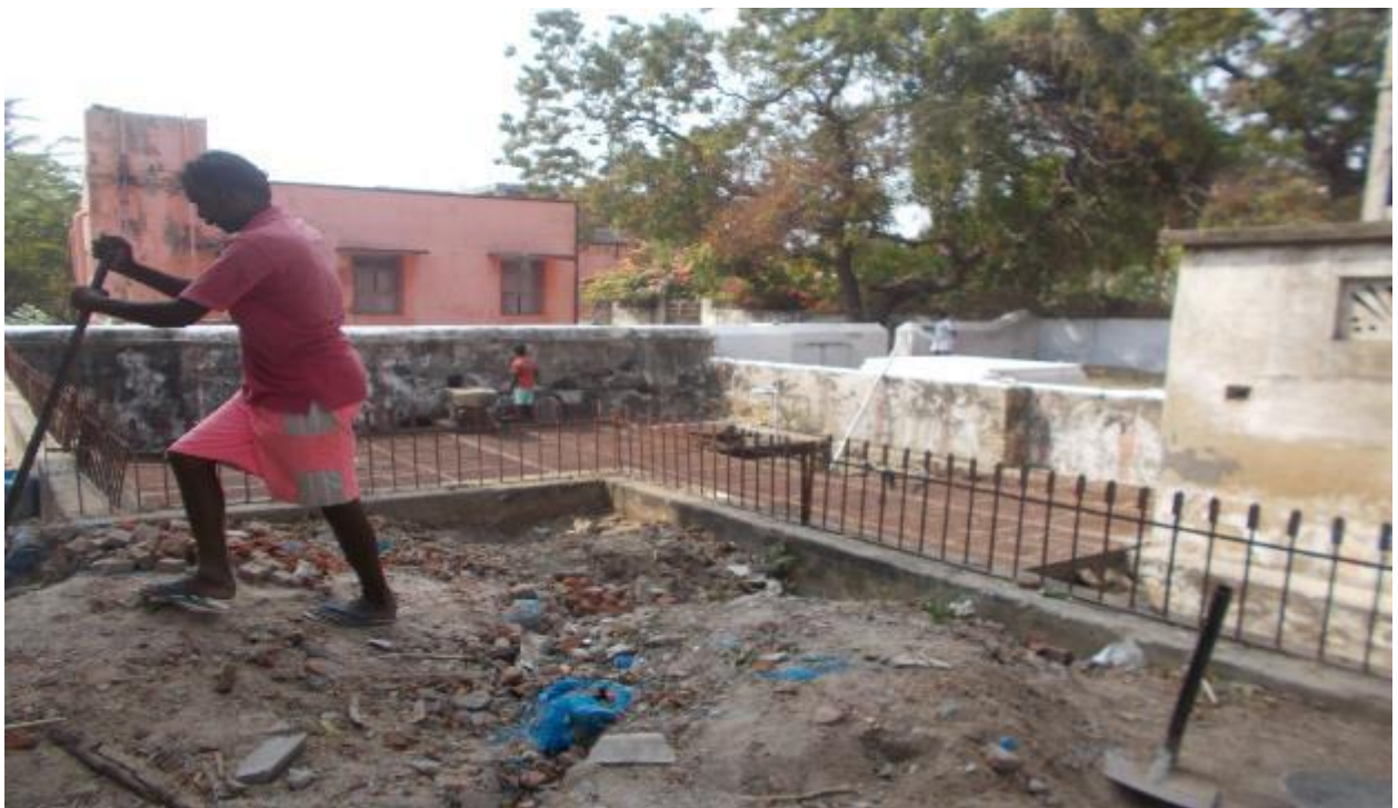
Wall being Raised
