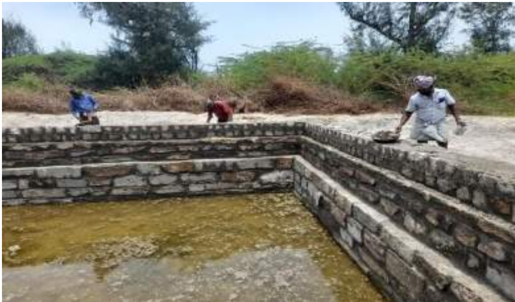
Raising the Parapet walls
