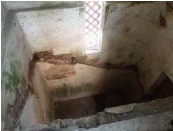
Collapsed Staircase
