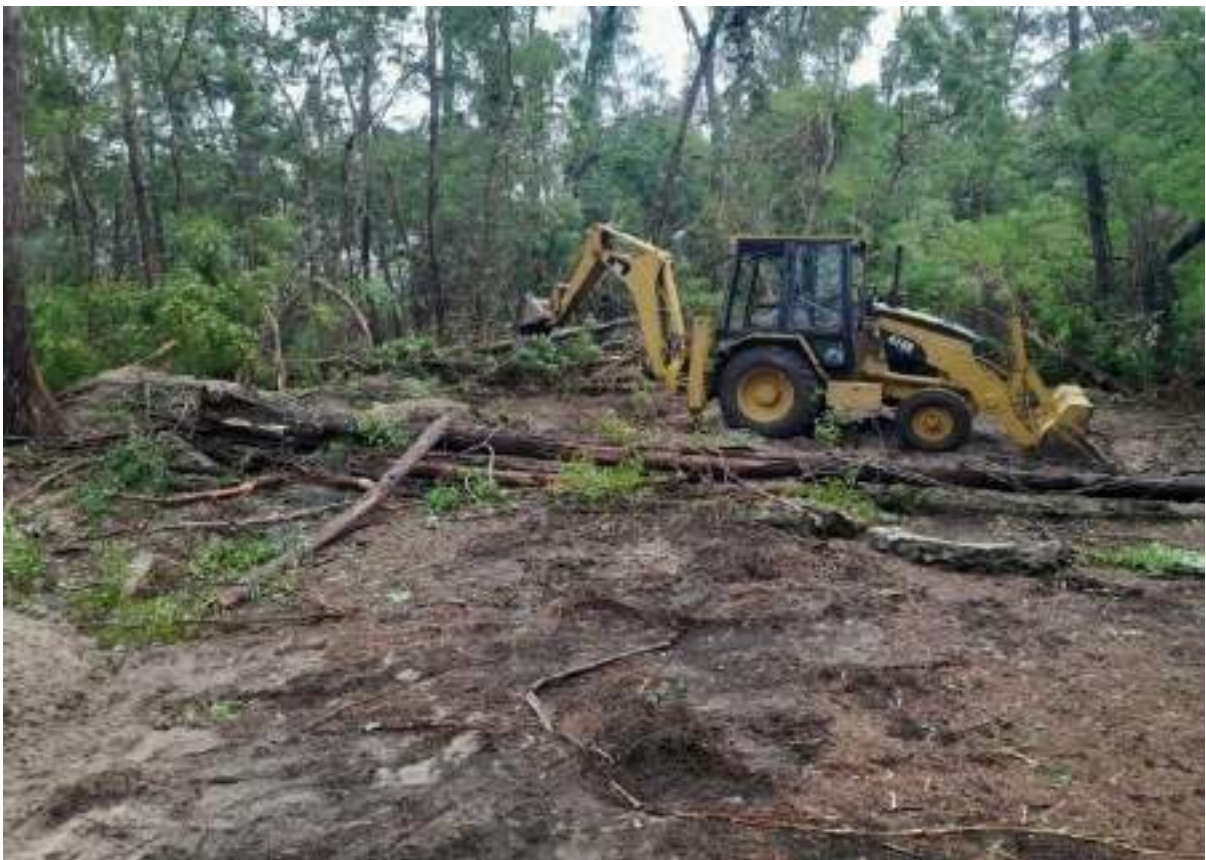
Thorny bushes being cleared by JCB
