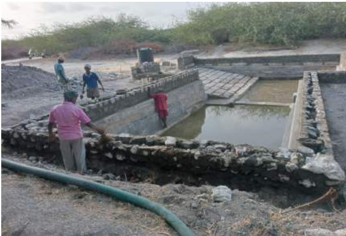
Construction of parapet wall is on...
