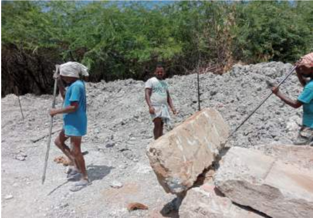
Recycling of material - old road side big stones, used for strengthening the traditional water body
