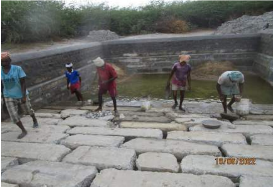
Another example of recycling of material:Huge paver blocks used for ramp
