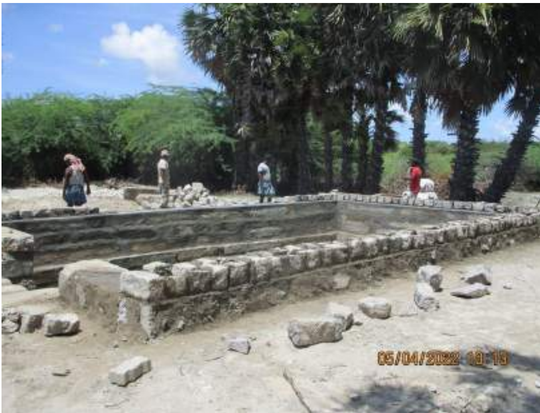
Raising the parapet wall
