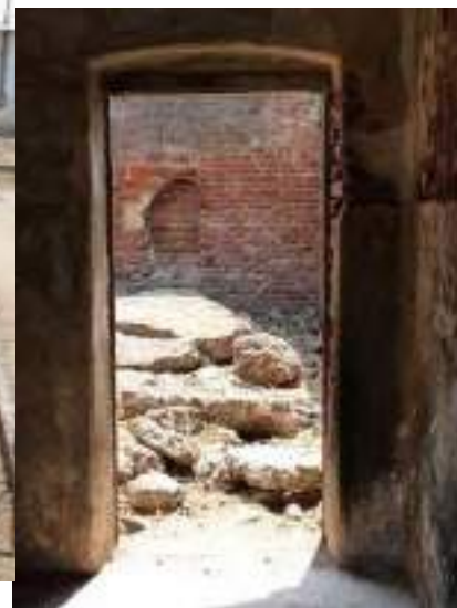
Collapsed Madras terrace roof
