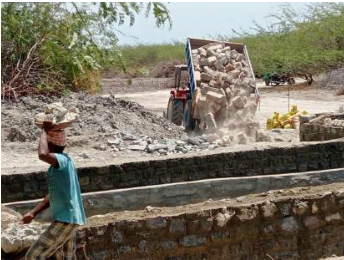
Transportation of good quality stones for constructing the wall
