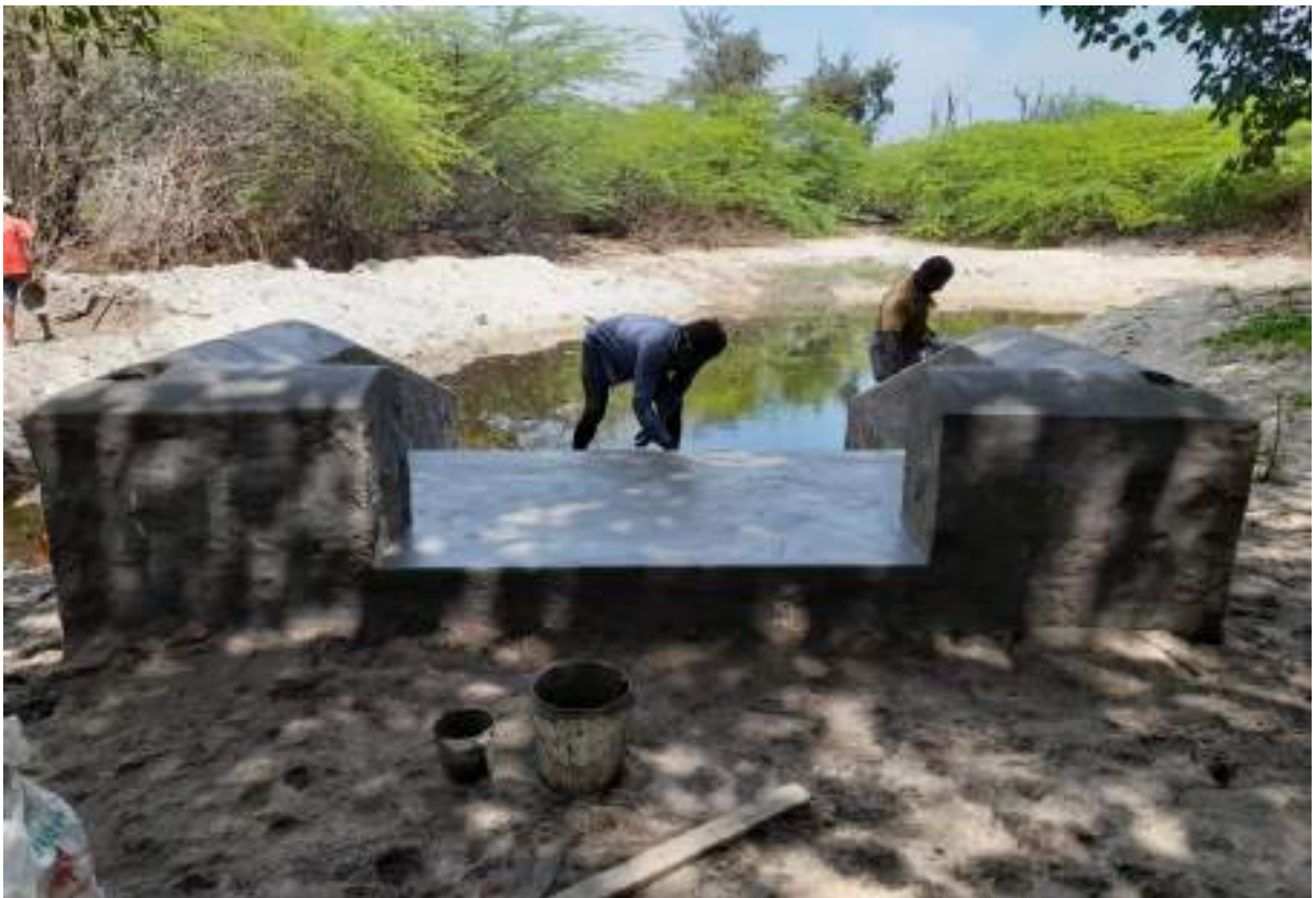
Construction of platform at the entry point
