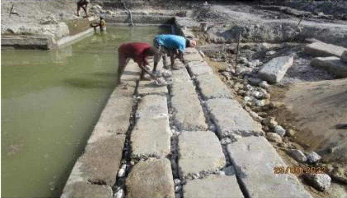
Strengthening the ramp
