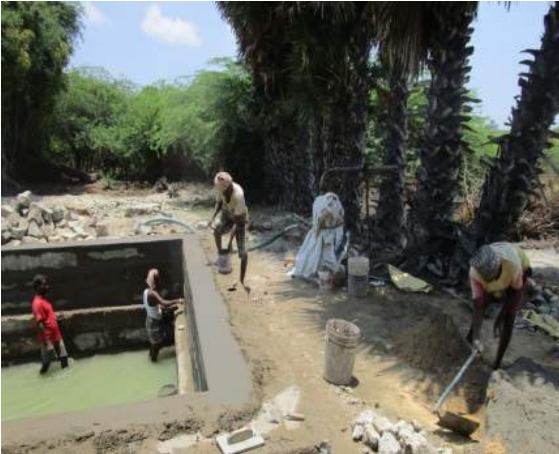
Construction work is on...A new Teertham is born
