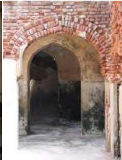
Deteriorated Plaster
