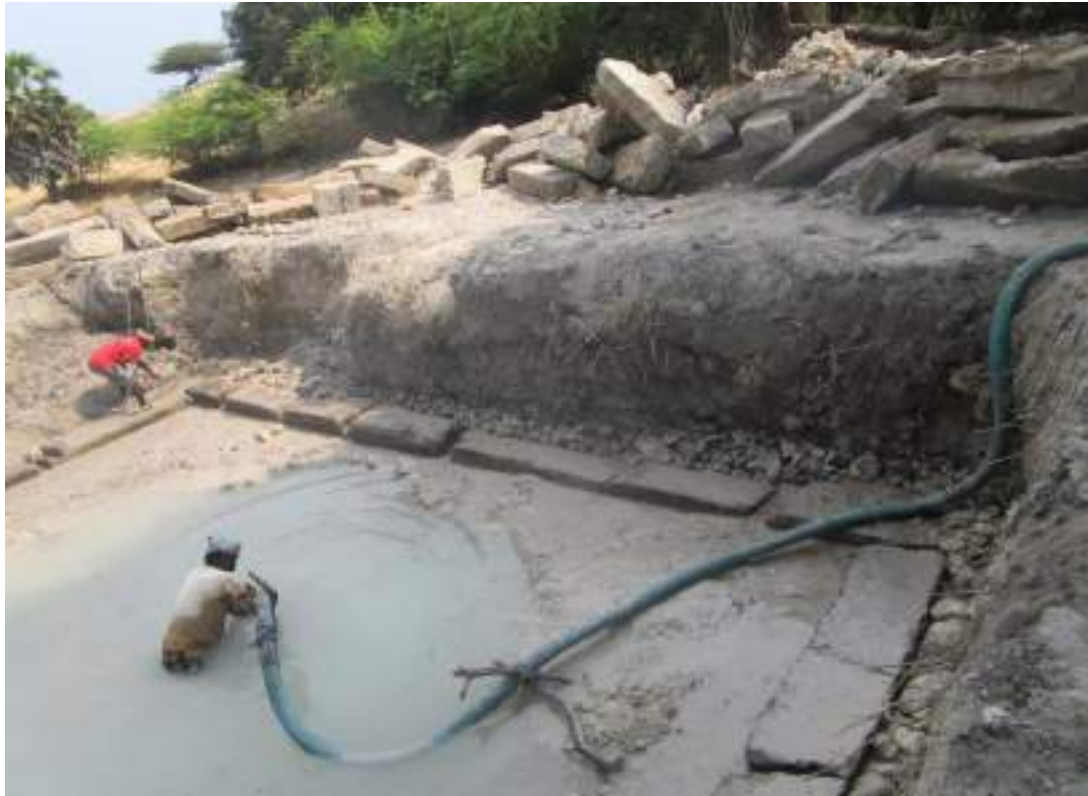
Pumping out the water after the initial excavation
