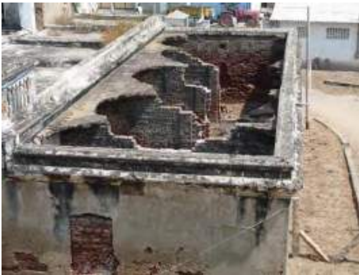
Collapsed Madras terrace roof
