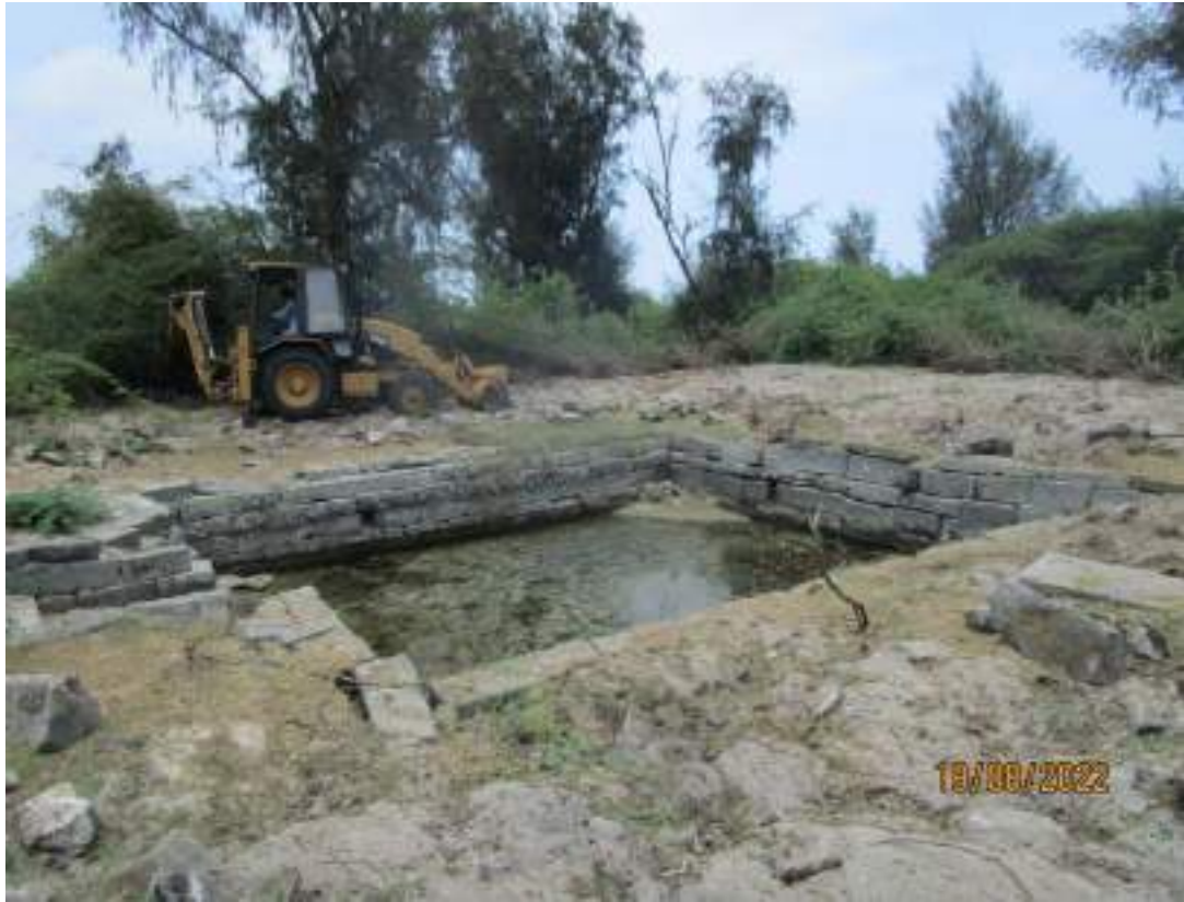
Clearing thorny bushes
