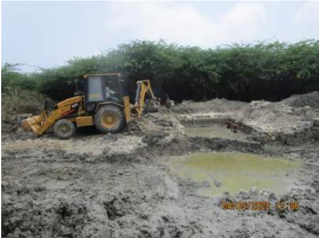
A JCB is doing the work at breakneck speed
