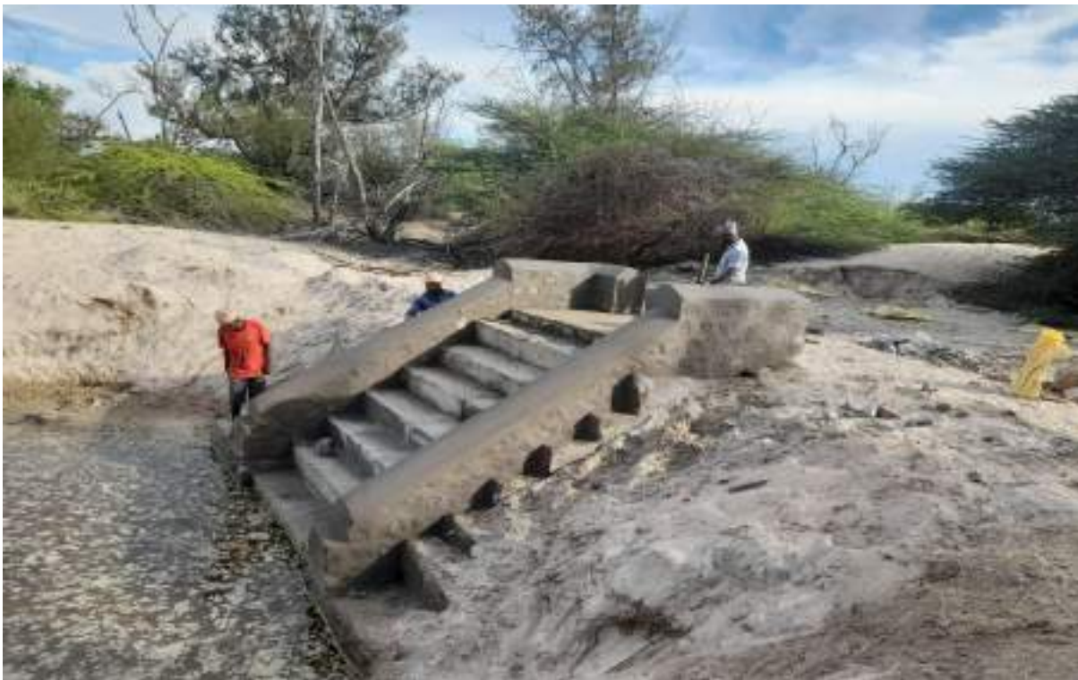
Construction of steps for easy access to the Teertham
