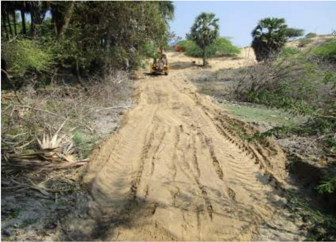
Laying the road to reach the Teertham site - 300 Meters
