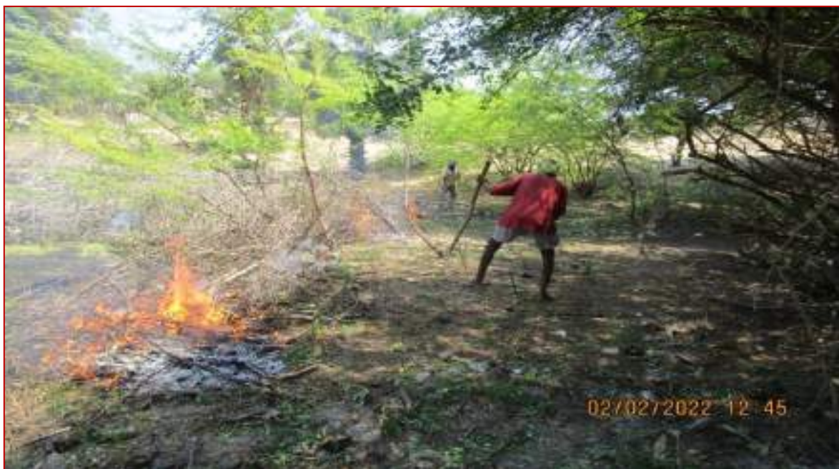
Removing the thorny bushes and debris
