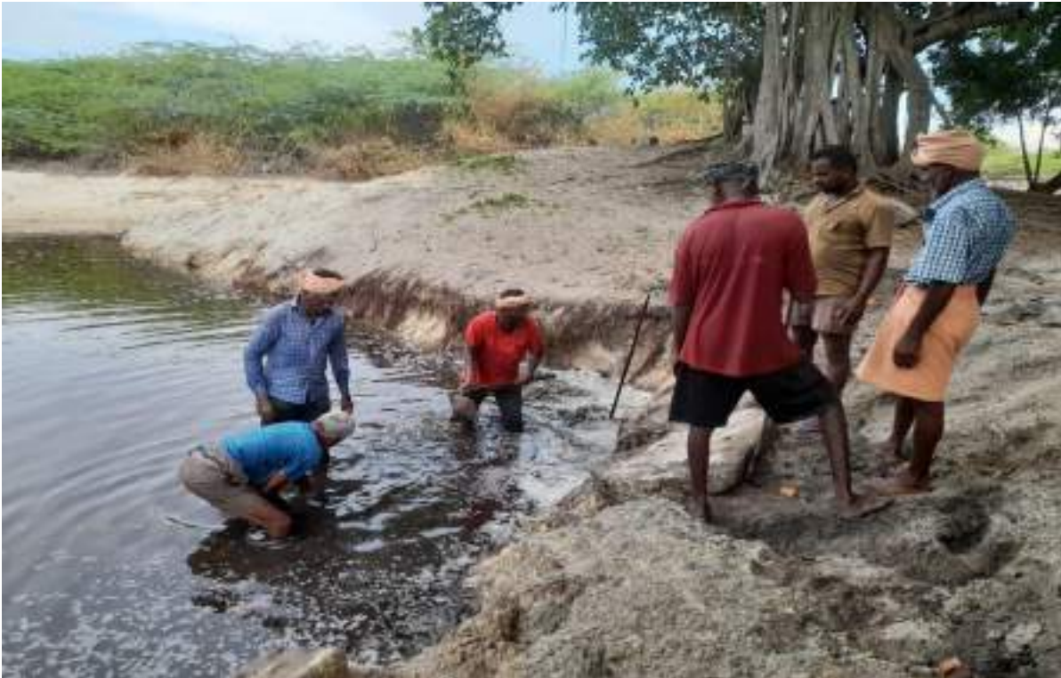
Cleaning of the dirt from the water body
