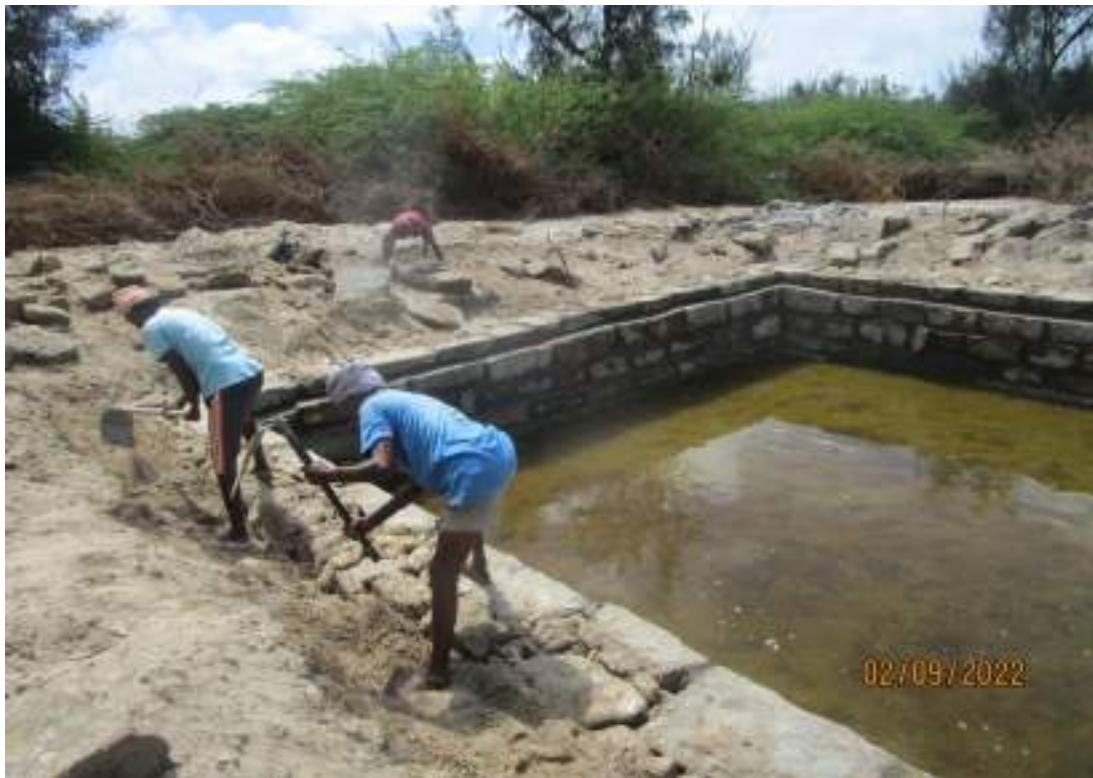
Strengthening Side walls
