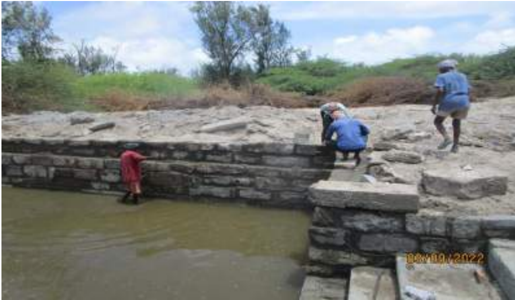
Repairing Sidewalls
