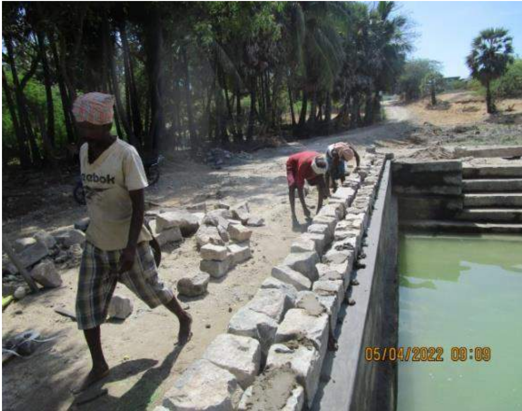
Construction of parapet wall...
