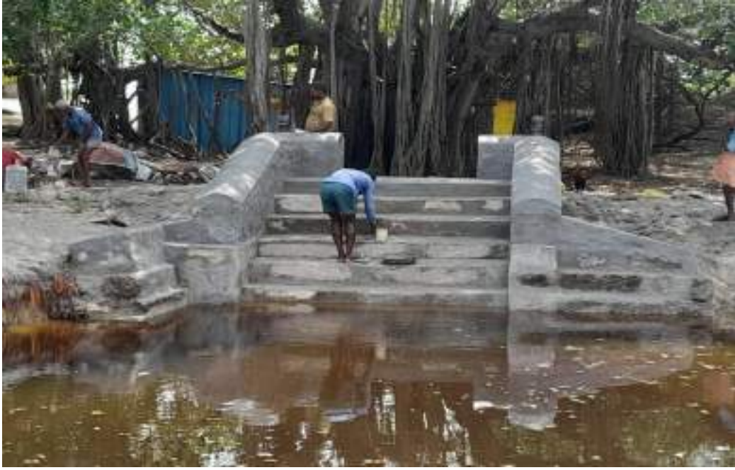
Steps under construction
