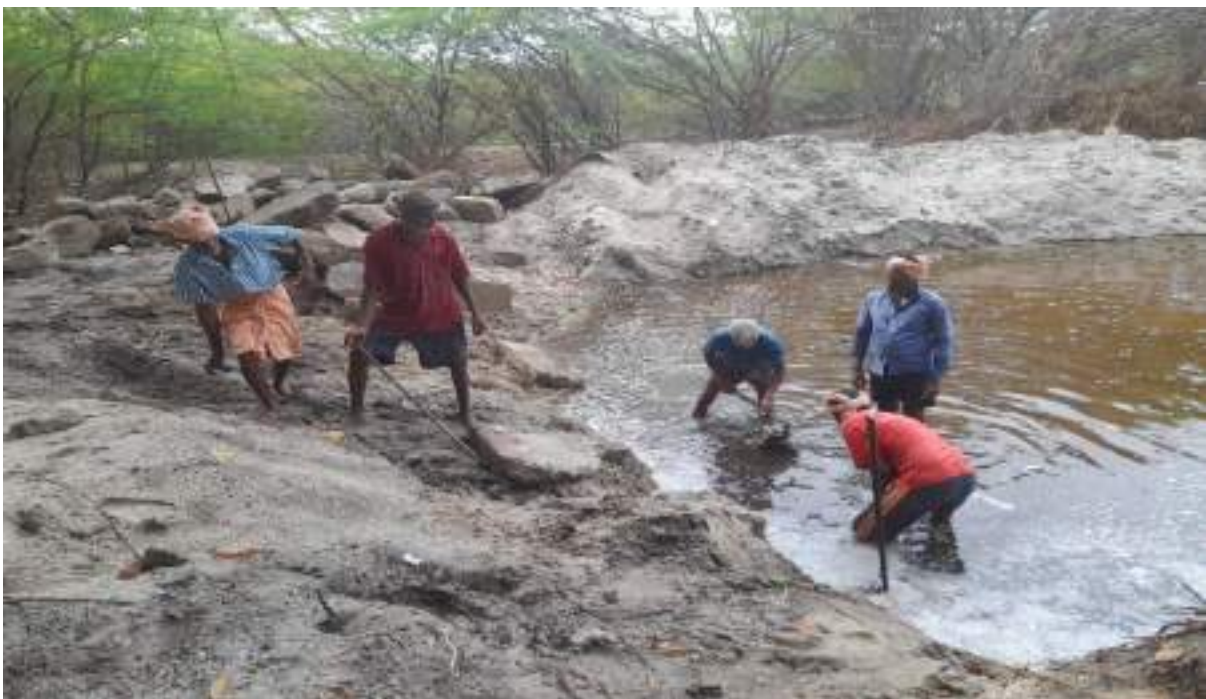
Water started oozing after digging only one foot
