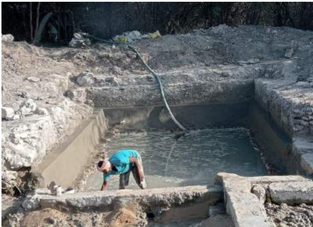
Plastering work is on ....
