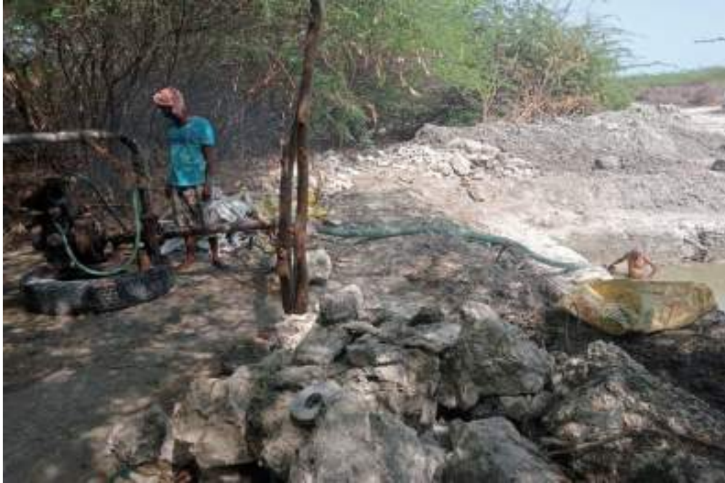
Pumping out the dirty water before desilting
