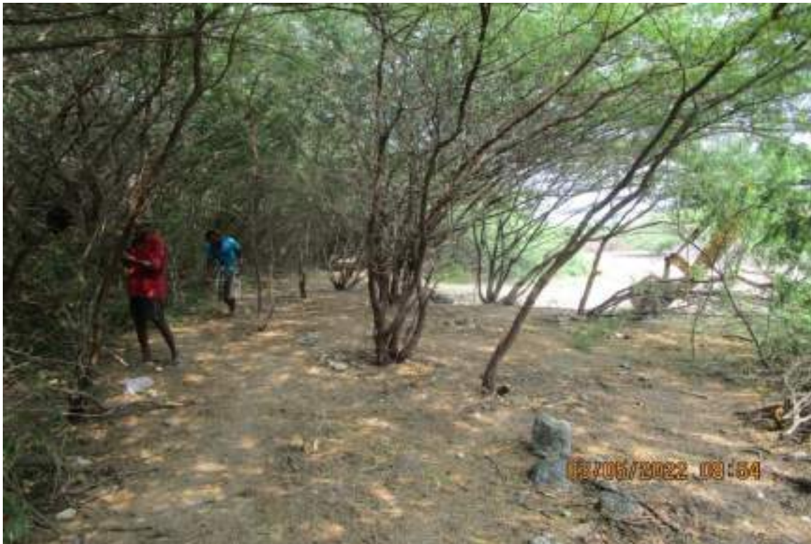
Clearing the area for free movement of JCB etc.
