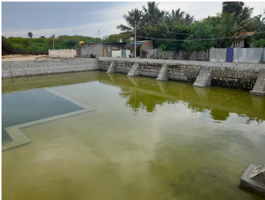
Beautiful view of Simha Teertham with piers holding the wall
