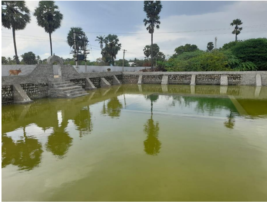
Another view with steps and entry gate
