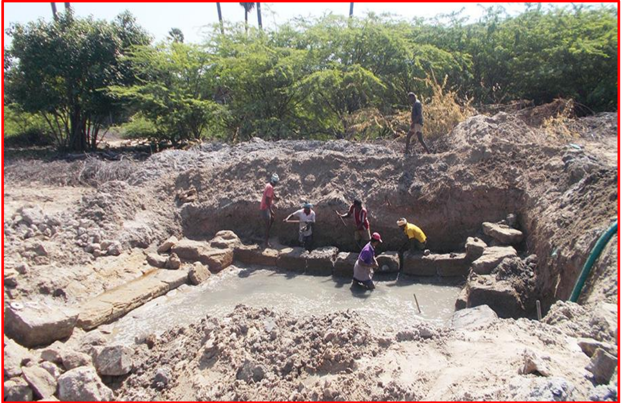
Pumping out the water and then laying the foundation stones
