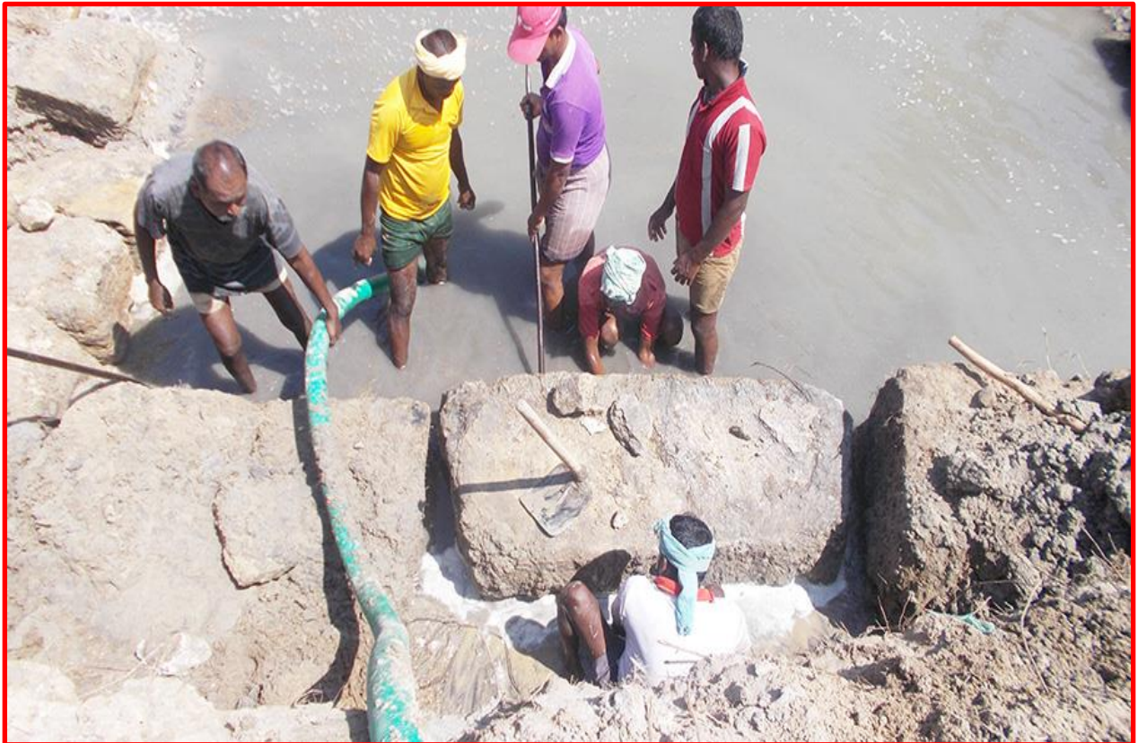
Pumping out the water and then laying the foundation stones
