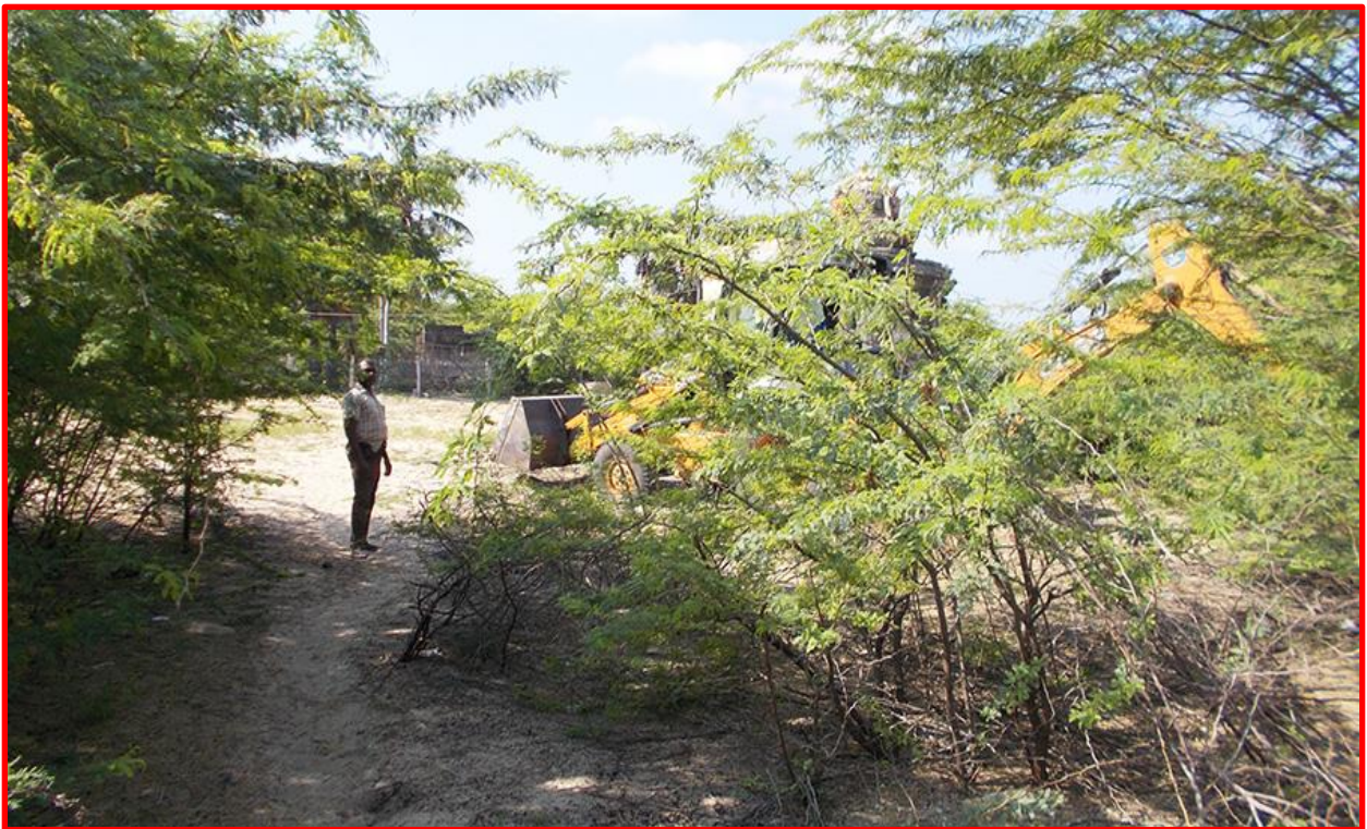
Cleaning and removing Odai trees at site with the help of machinery and manually
