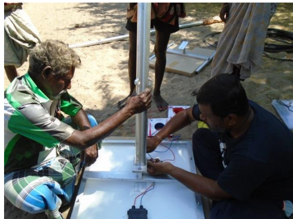
Shri.Raghu of Sairam solar installing the
