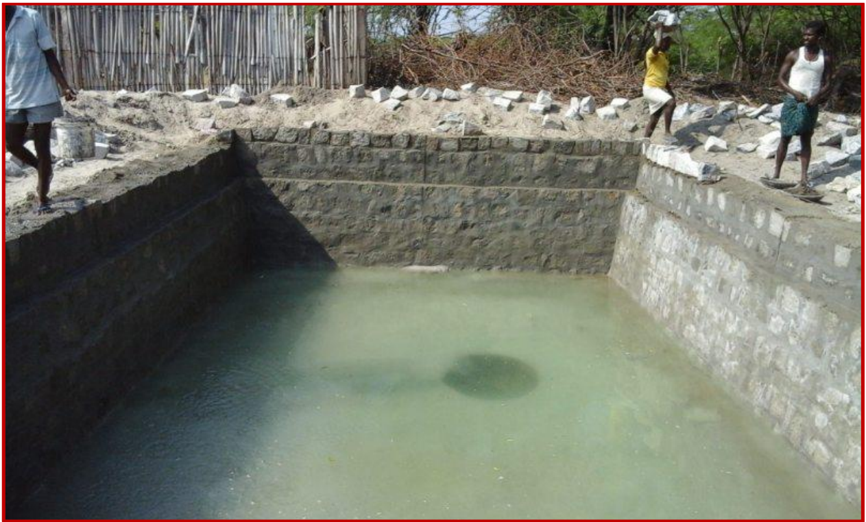
Work of side steps and retaining wall is on ...
