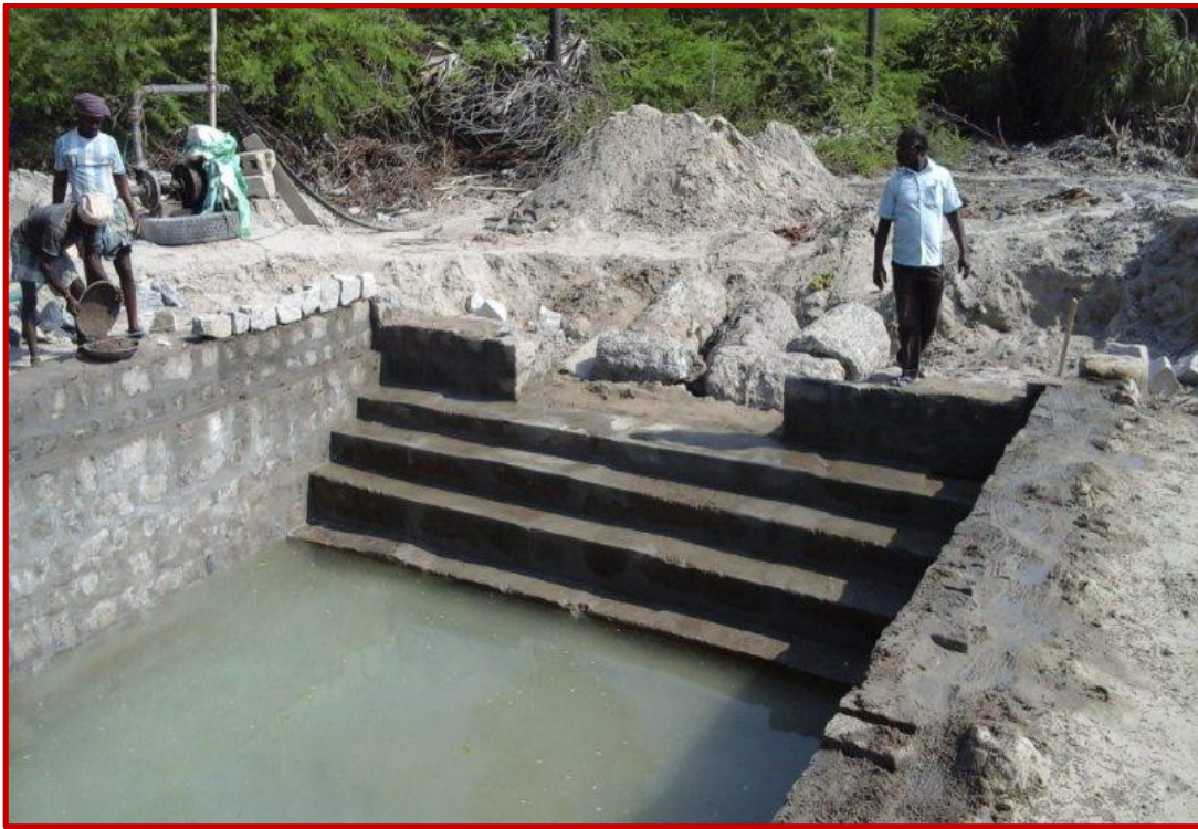
Shri.Kadiresan, Supervisor at site inspecting the work
