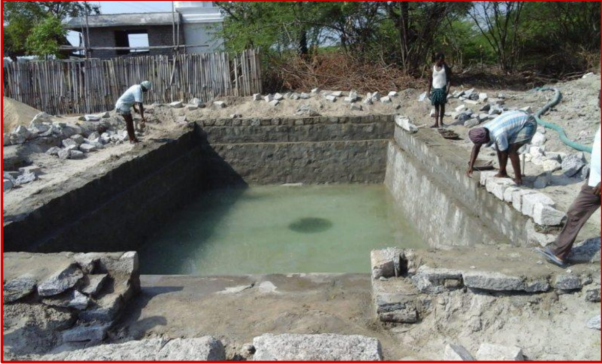
Construction of side wall is in progress ...
