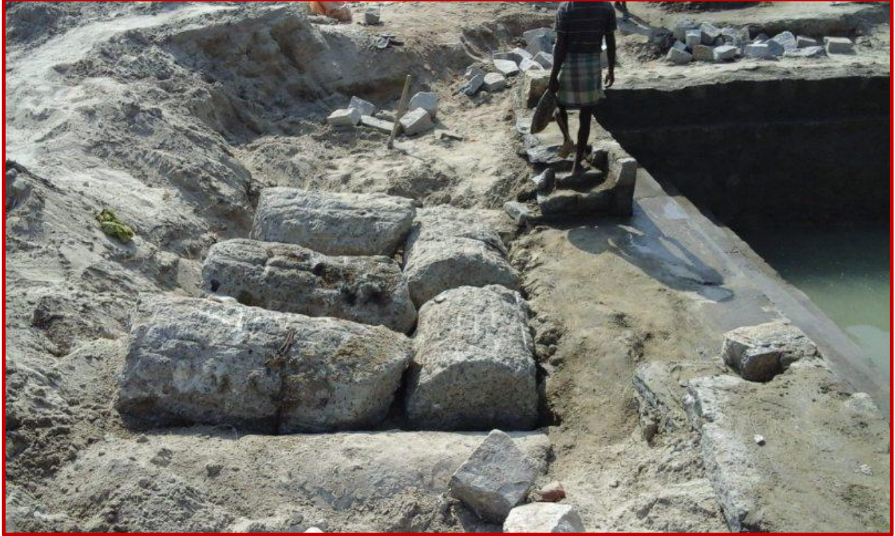
Huge concrete blocks brought from the nearby site to strengthen the structure
