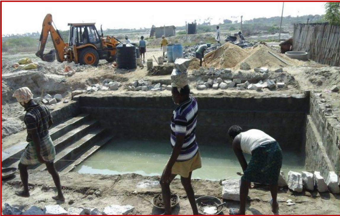
Construction of side wall is in progress ...
