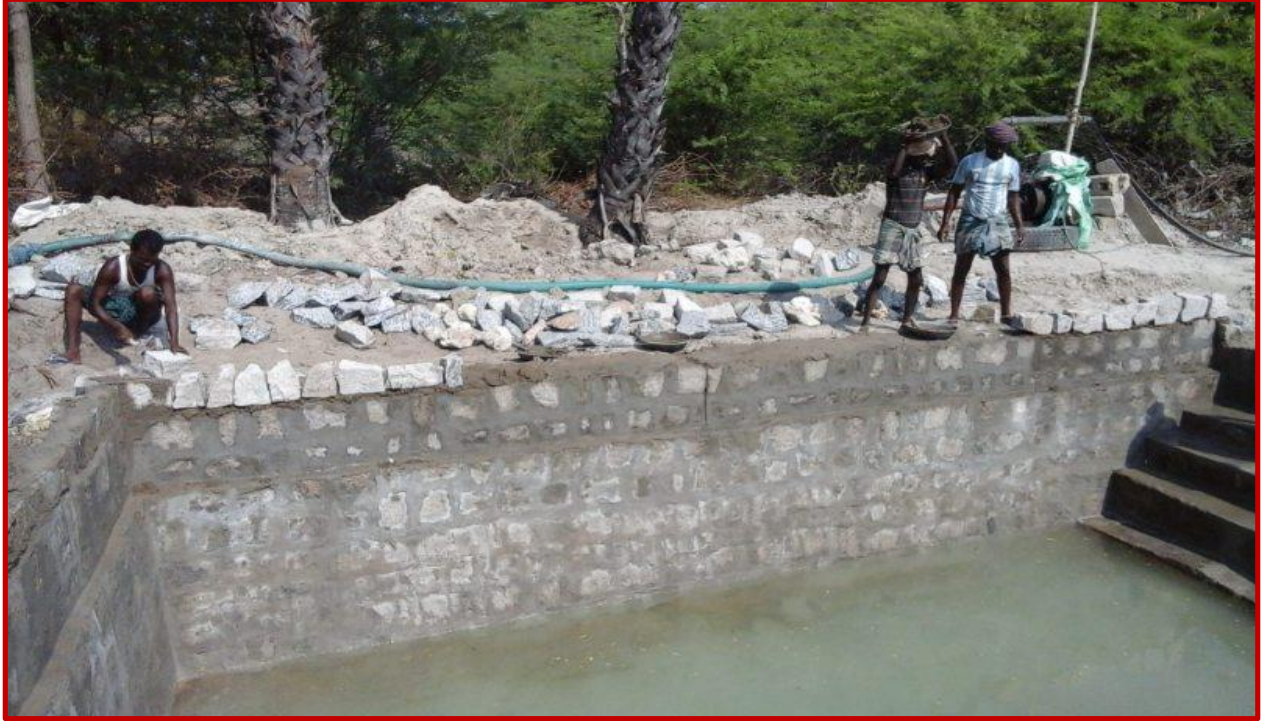
Work of side steps and retaining wall is on ...
