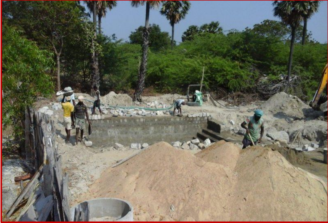
Pumping the water for constructing the bed
