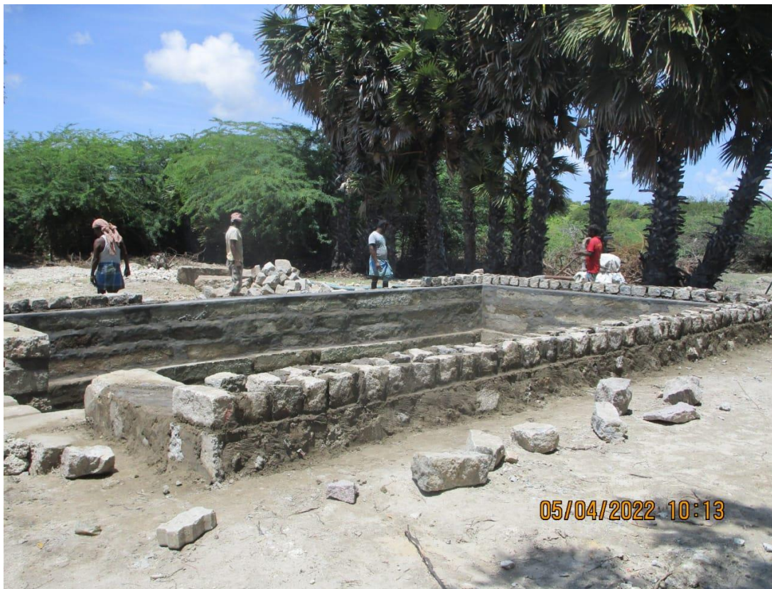
Construction of parapet wall ....
