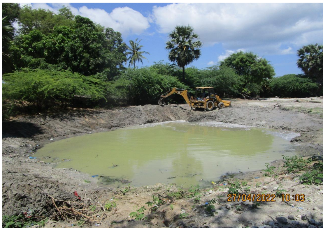
Levelling of the area and bunding to give proper shape to the water body
