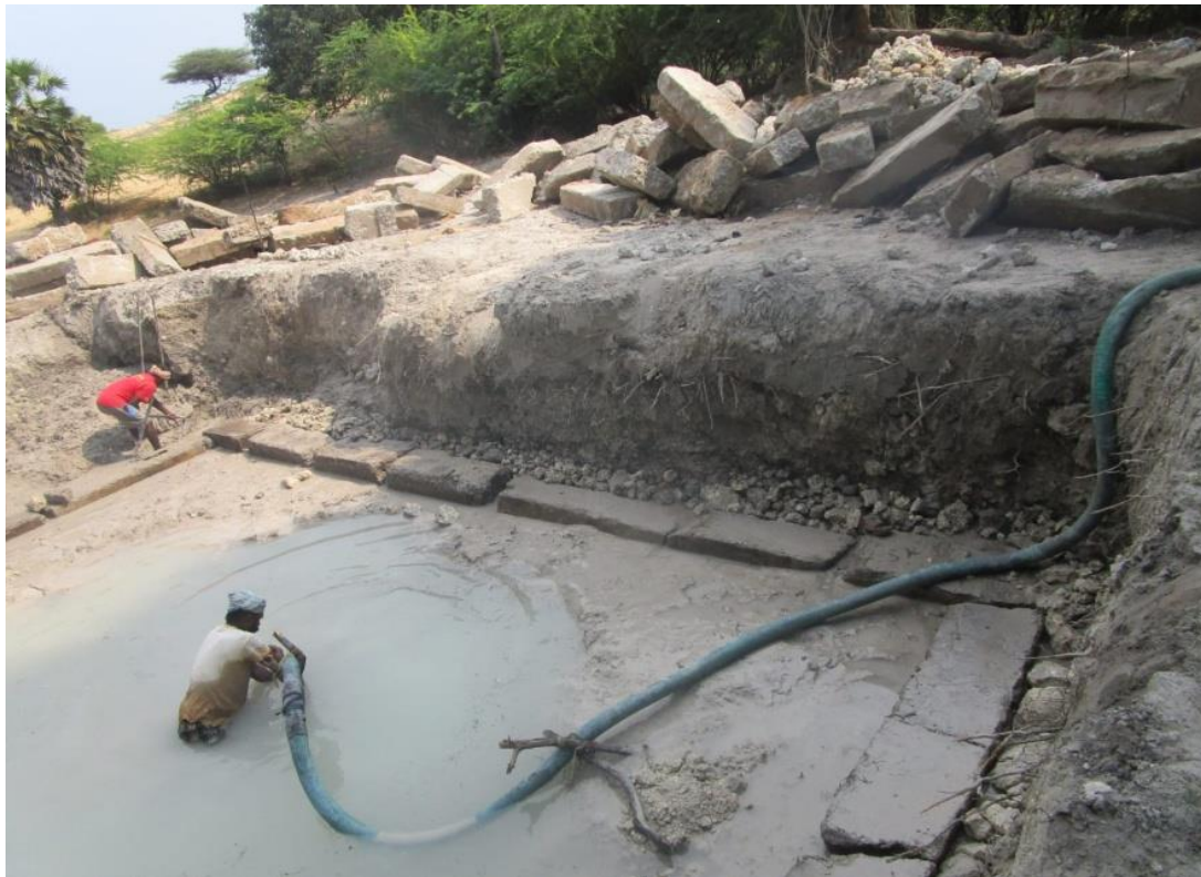
Pumping out the water for further construction
