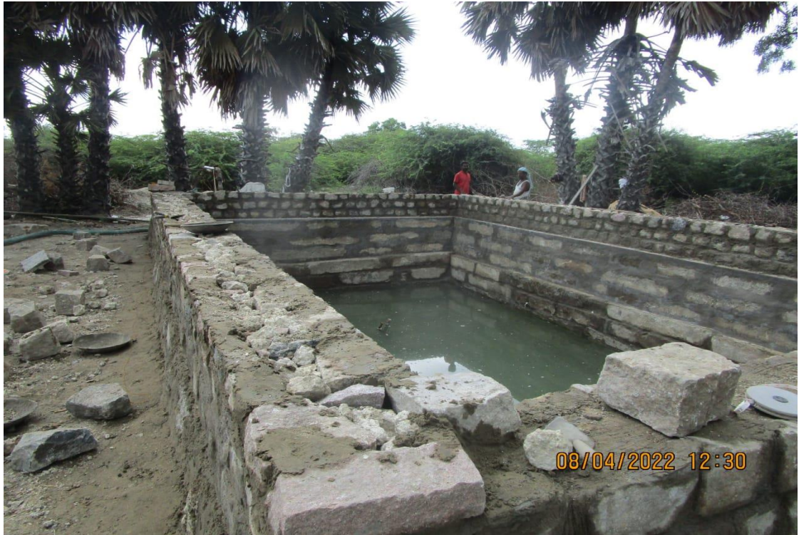
Giving finishing touches by sloping the top portion and cementing it
