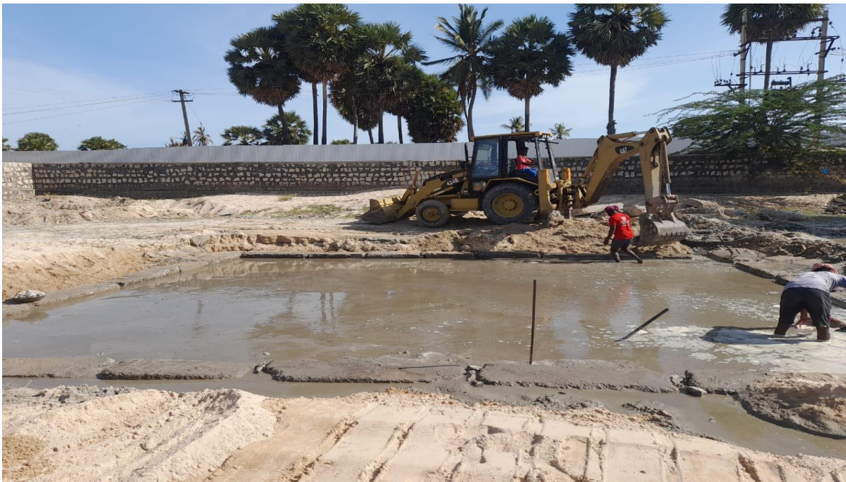
Construction of inner pond has started
