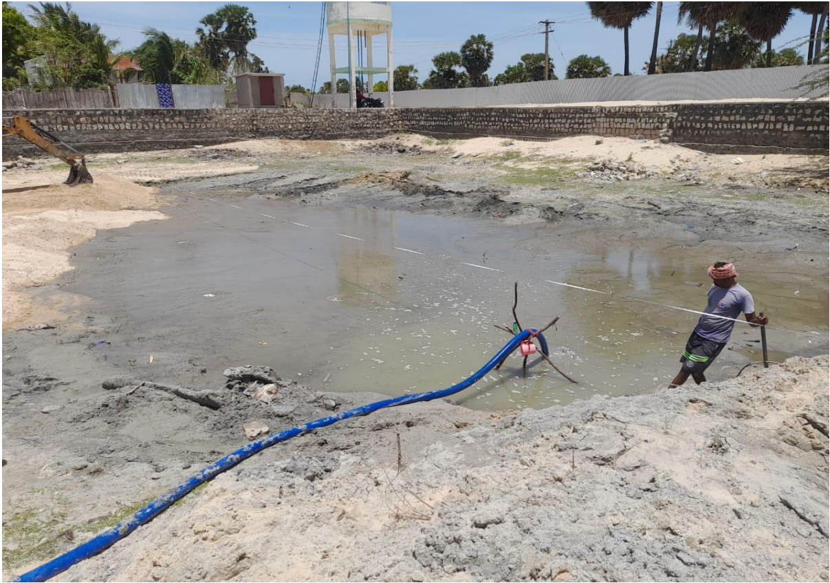
Pumping out the water before marking the boundaries of inner pond
