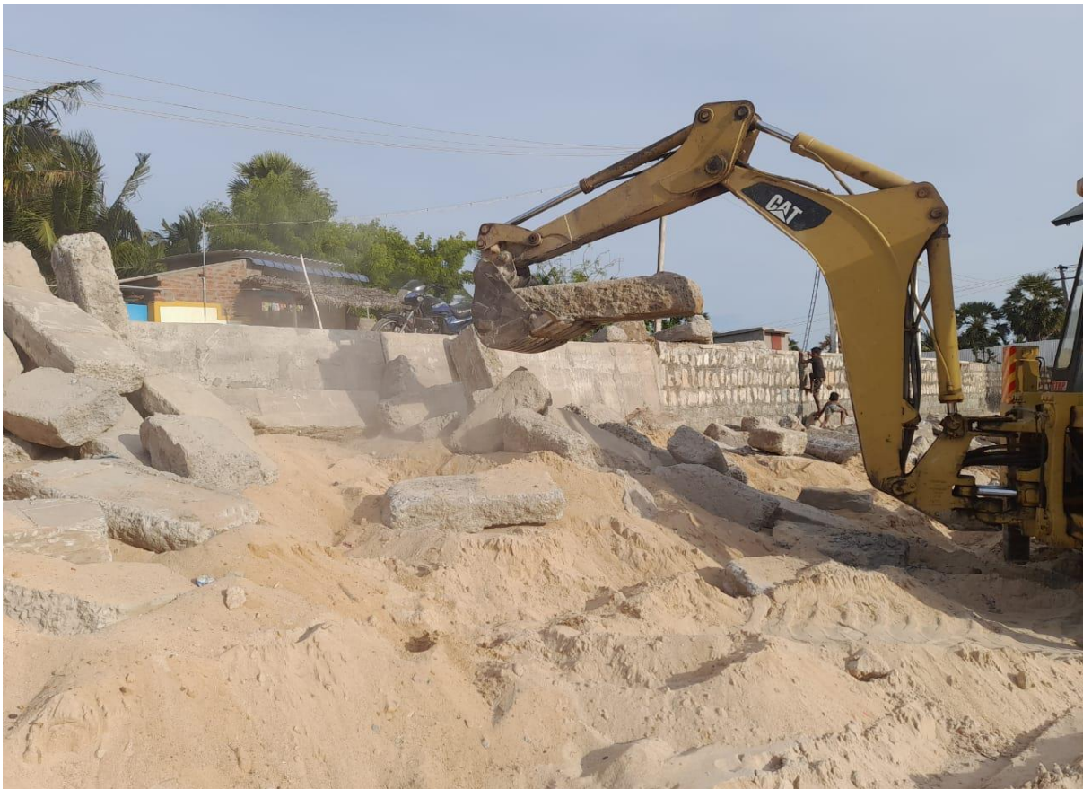
Bigger size stones for the basement moved with the help of JCB
