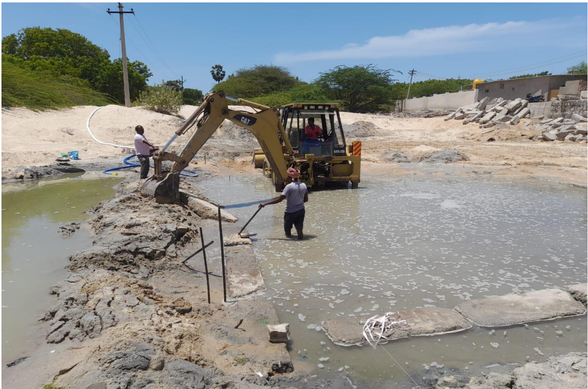
JCB at work for placing the stones of inner pond
