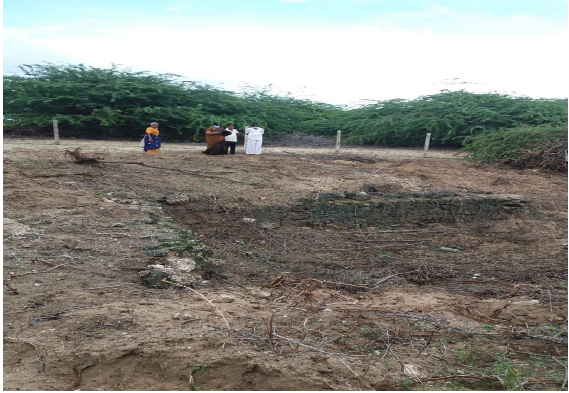
Gaja Teertham site getting ready for renovation
