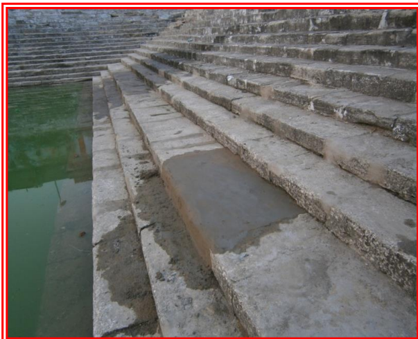
All the steps were repaired and fresh sand spread in the tank to avoid growth weed
