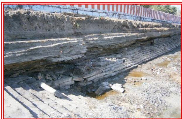
Damaged side walls full with vegetation and broken steps
