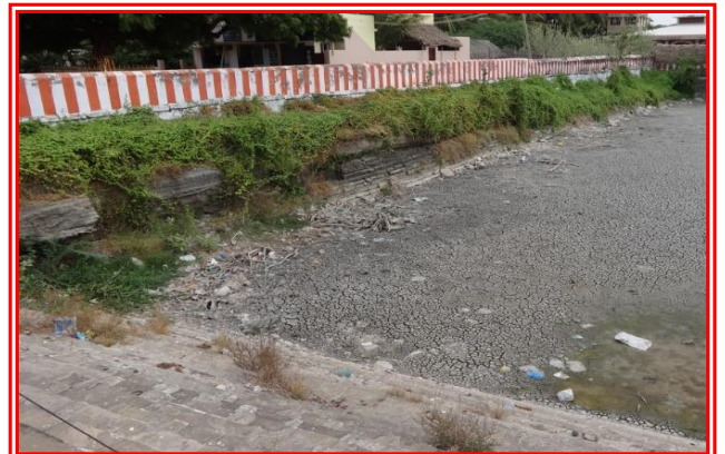
Damaged side walls full with vegetation and broken steps
