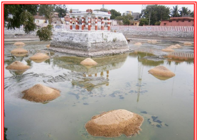
All the steps were repaired and fresh sand spread in the tank to avoid growth weed
