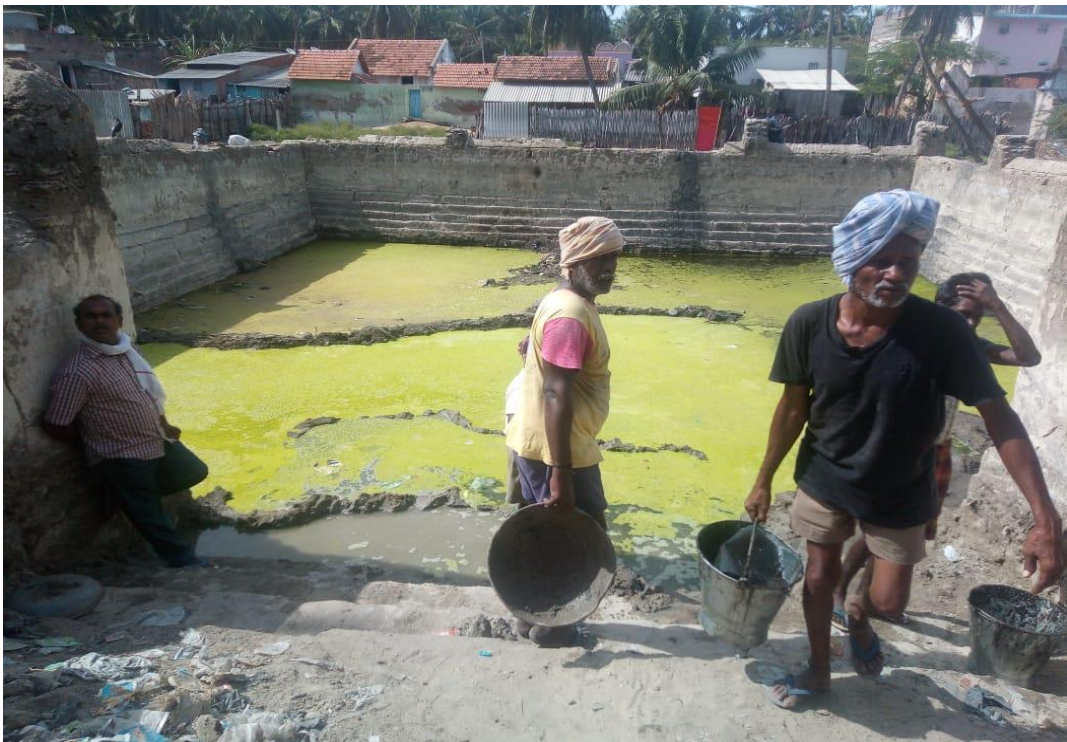
Putrefied water body – workers removing tons of mud manually
