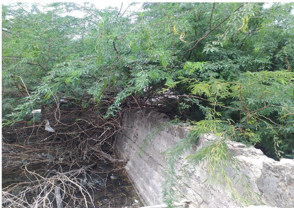
Condition of TWB before starting the work
