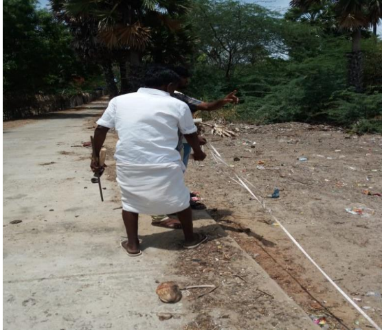
Near Bhima Teertham markings before the start of the cleaning
