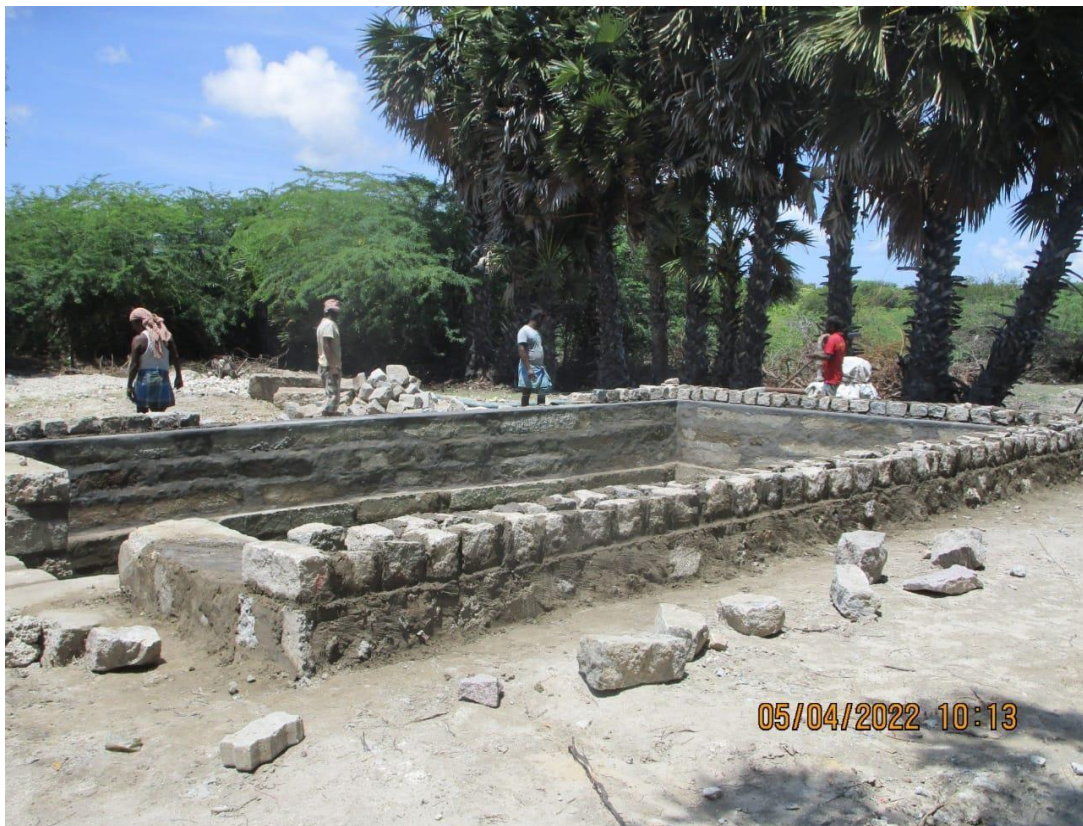
Raising the parapet wall
