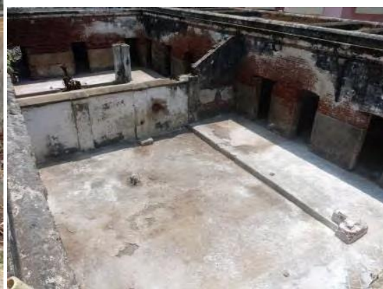
Damaged passage roof
