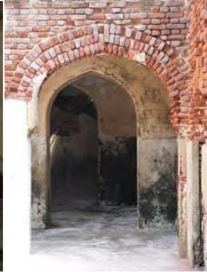
Deteriorated Plaster
