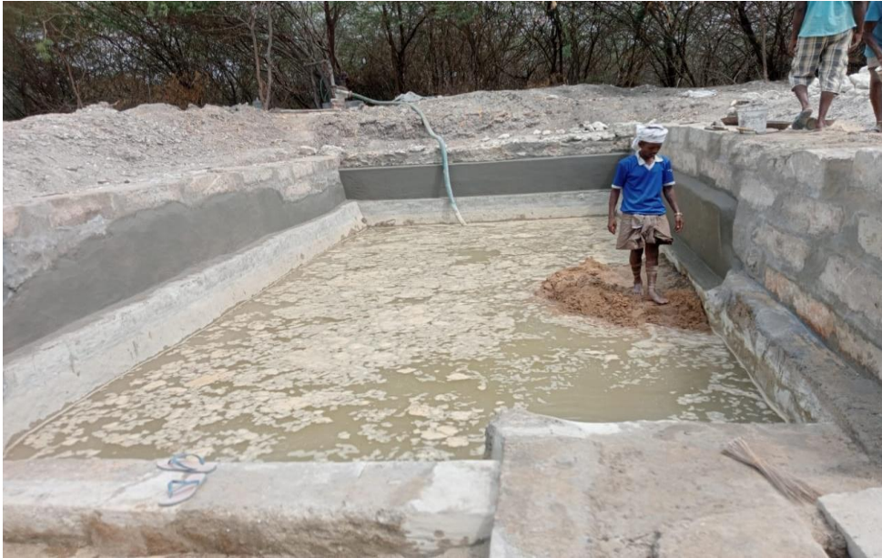
Spreading of sand - \frac{1}{2} feet throughout the Teertham base for better maintenance
