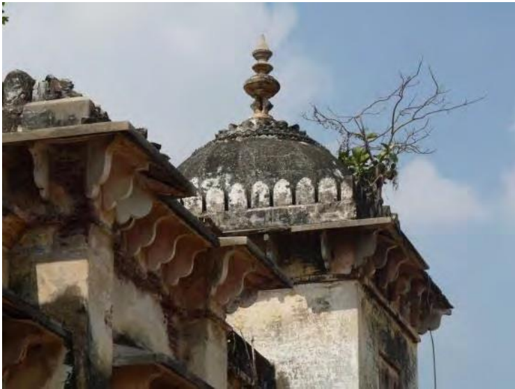
Condition of the domes - full of vegetation and cracks
