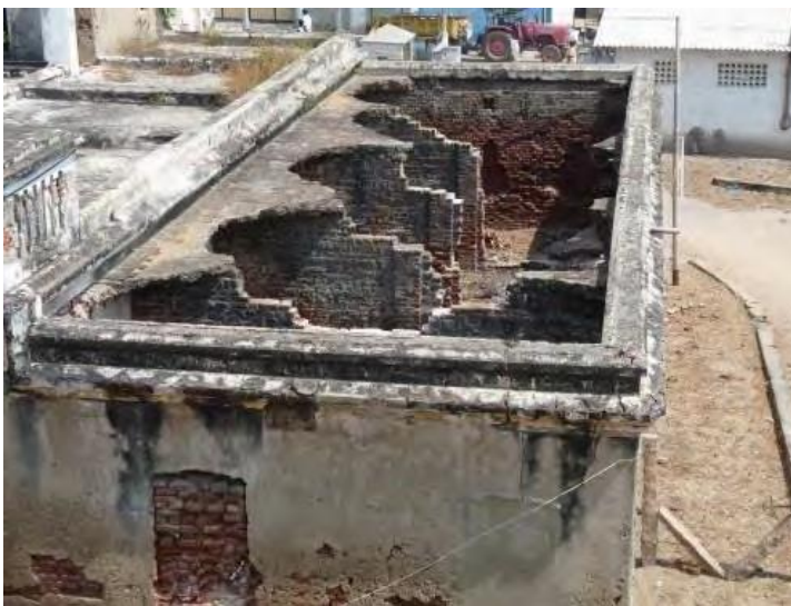
Collapsed Madras terrace roof
