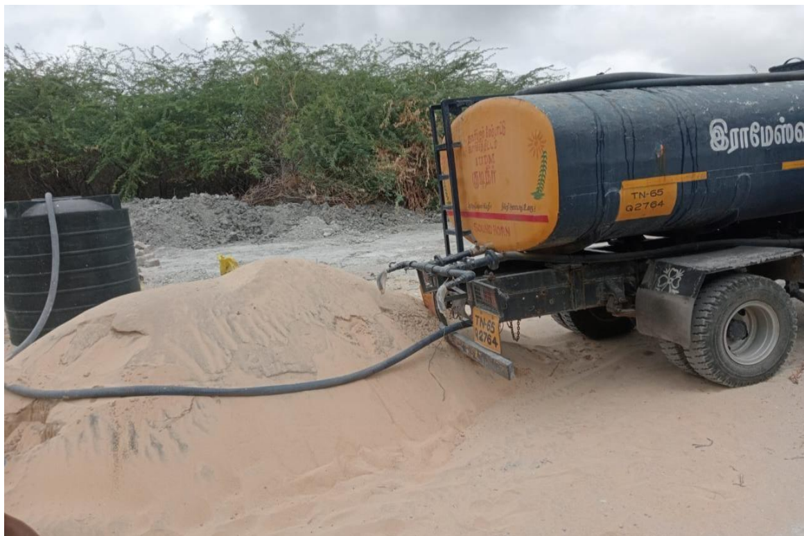
Good, fresh water is brought in a tanker for construction work as the local water is saline
