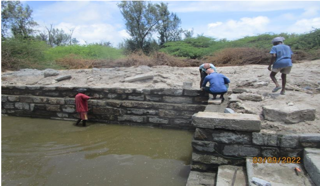
Repairing Sidewalls
