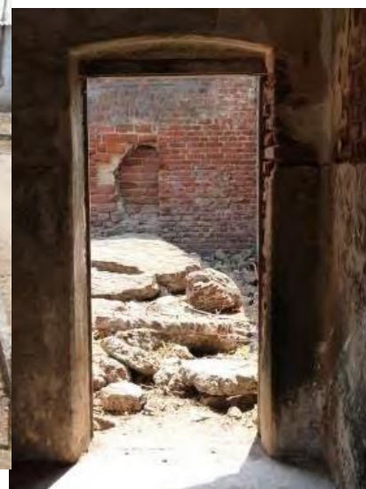
Collapsed Madras terrace roof
