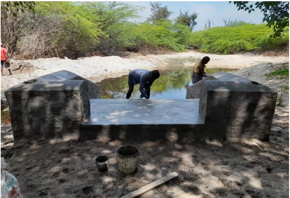
Construction of platform at the entry point
