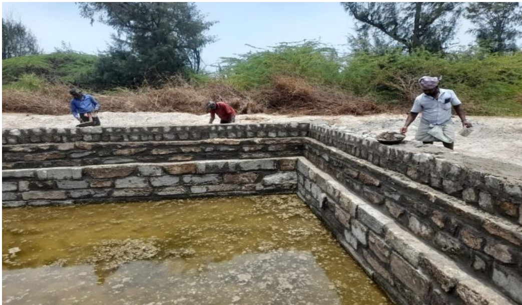
Raising the Parapet walls
