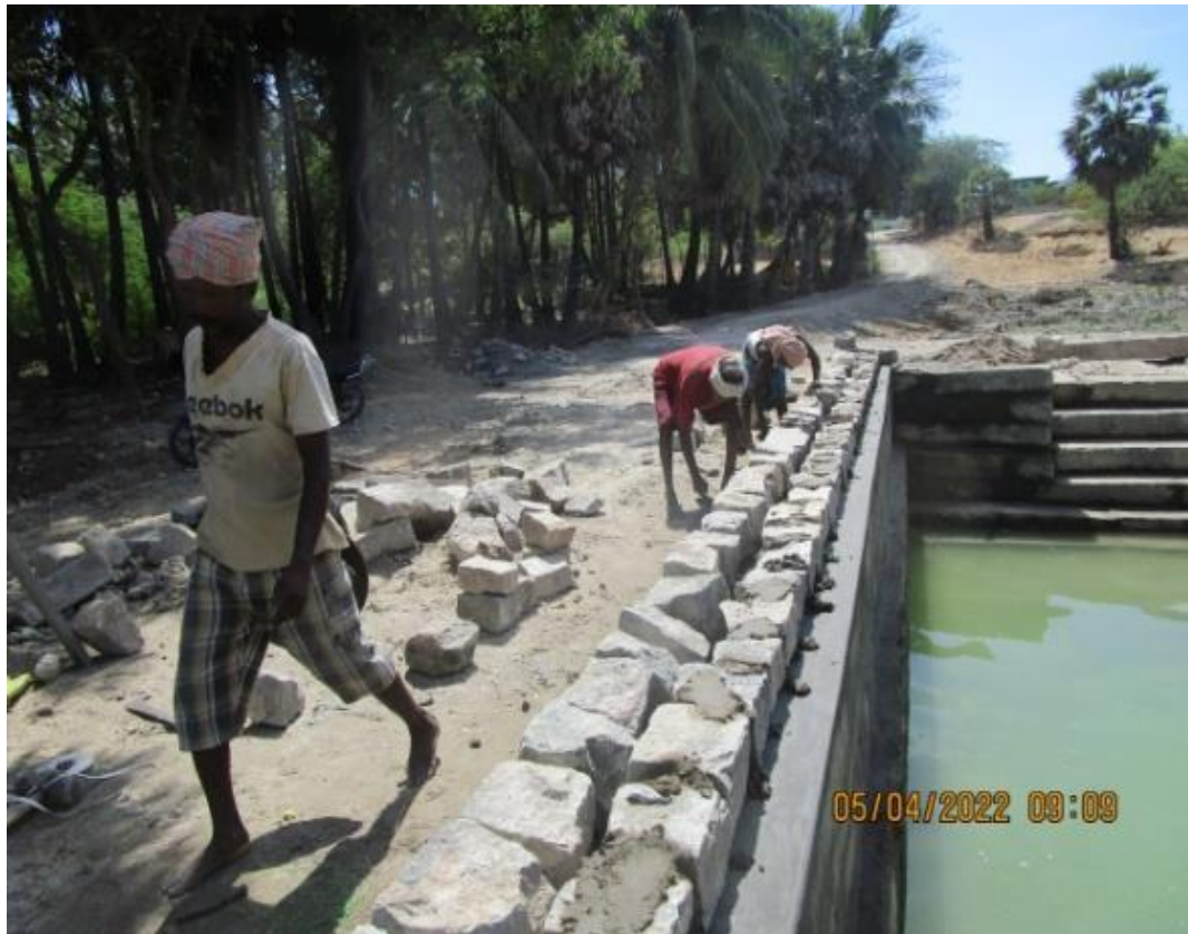
Construction of parapet wall....
