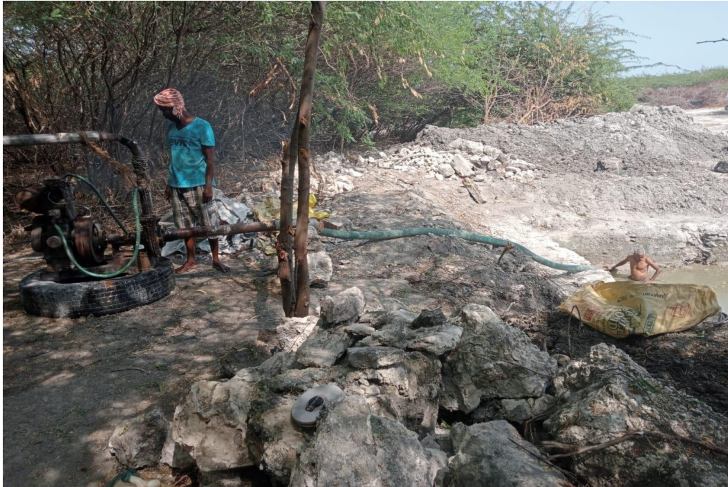
Pumping out the dirty water before desilting
