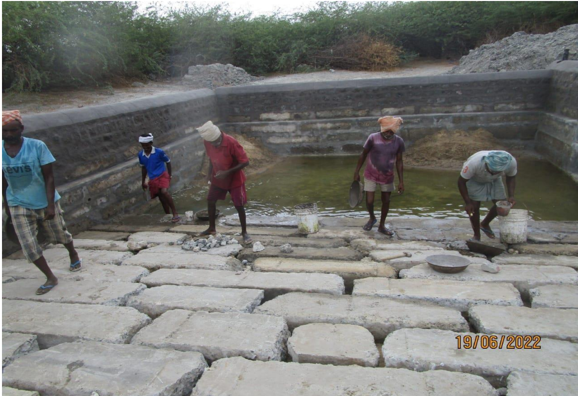
Another example of recycling of material:Huge paver blocks used for ramp
