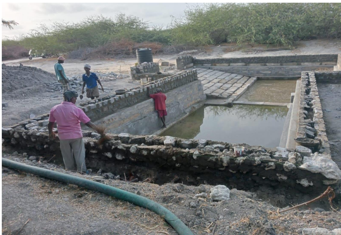
Construction of parapet wall is on...
