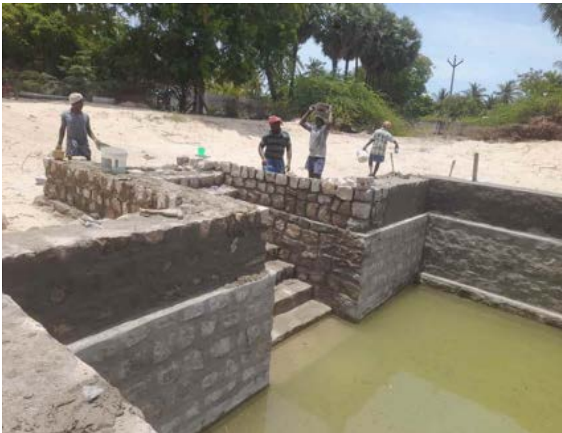
Construction of entry point and steps to the inner pond - also view the outer wall
