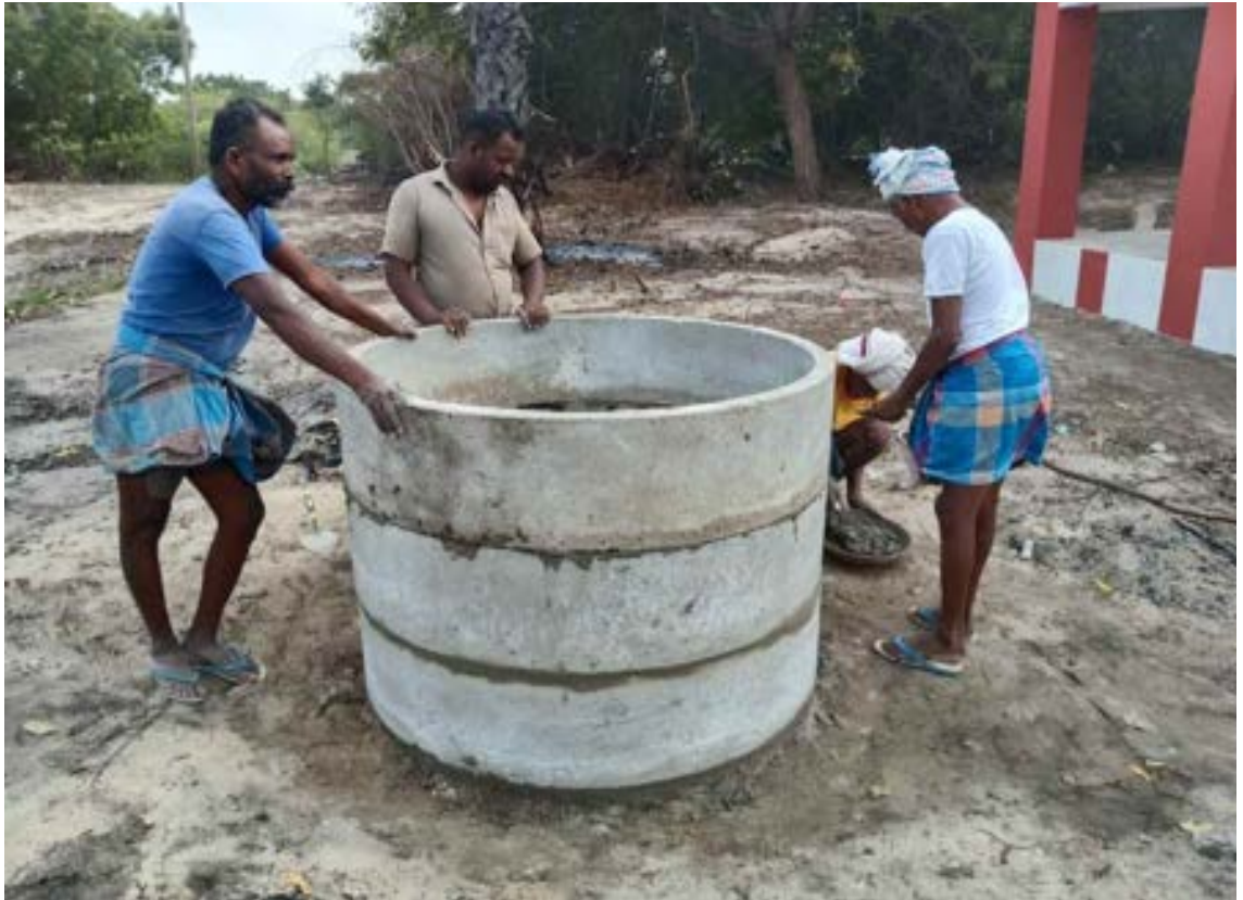
Ring well outside the Teertham which will be useful to the stakeholders as water has started percolating in it
