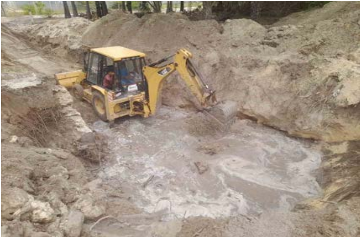
Dredging - deepening of the water body after removing the top layer of the dirt
