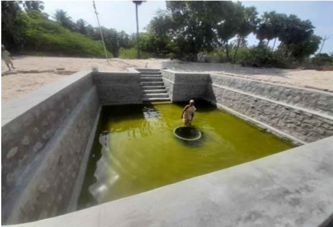
Ring well inside the inner pond which can be used during summer
