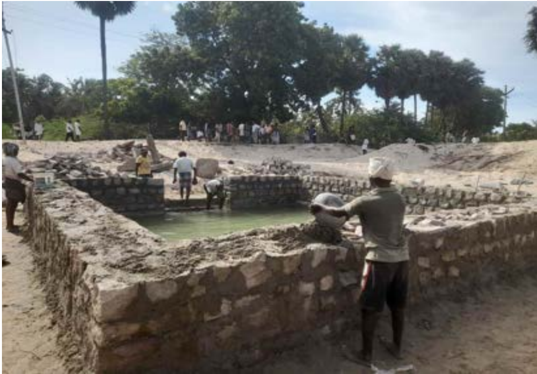
Increasing the height of the inside pond
