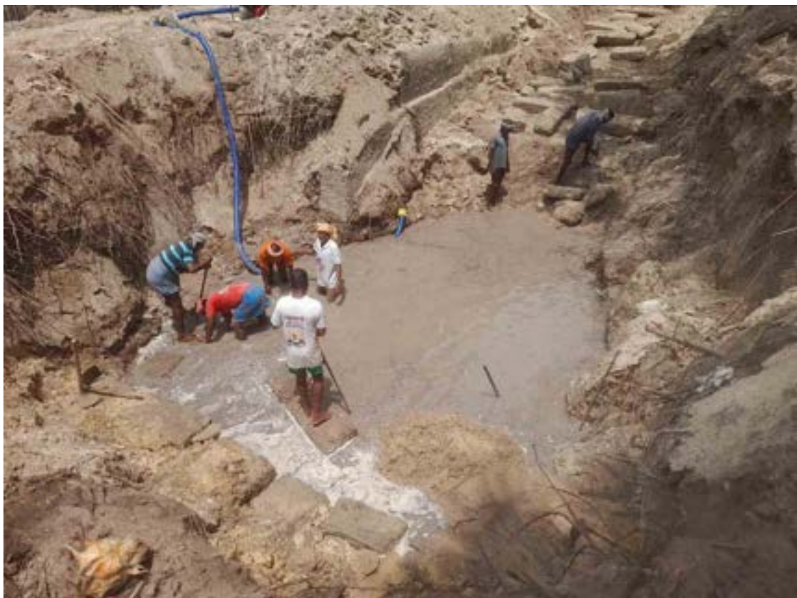
Workers putting the foundation stones after marking the area
