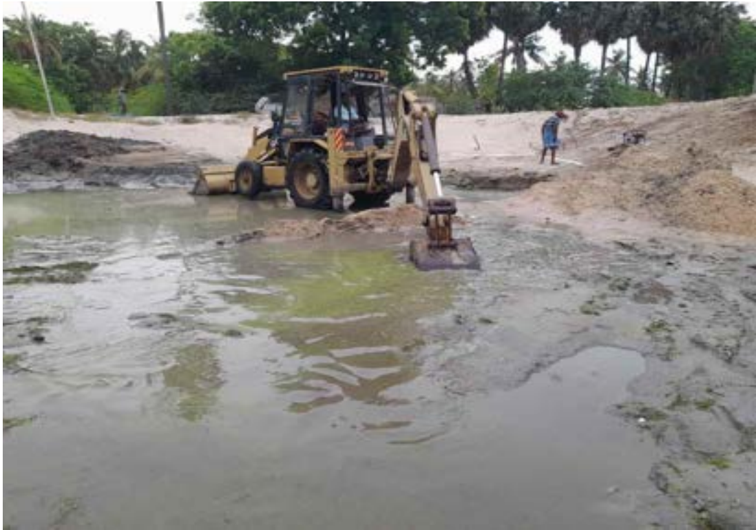
Use of JCB for desilting
