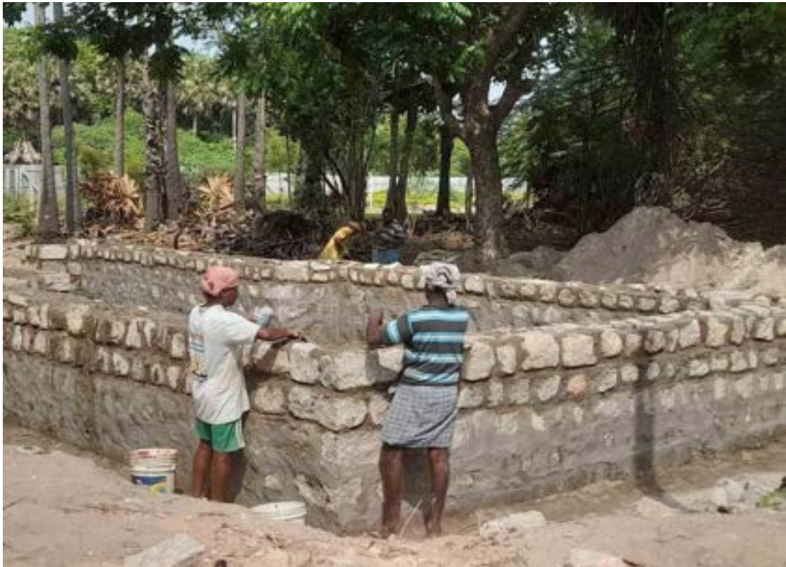
Raising the parapet wall to avoid sliding of mud and dust
