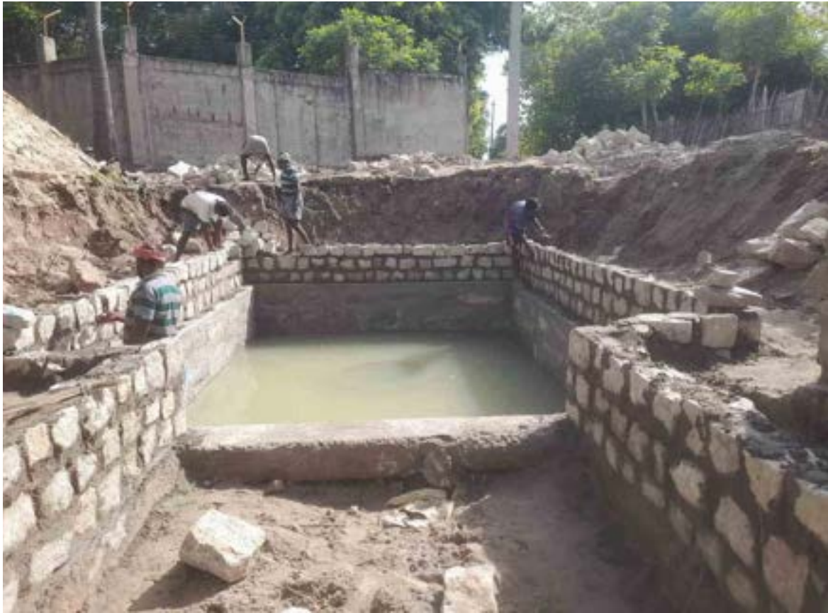
Increasing the height of the traditional water body
