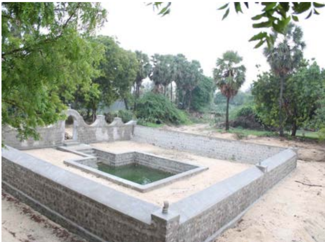
Complete view of both the inner and out ponds after plastering and pointing work
