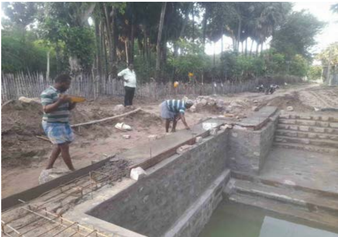
Strengthening the top portion by way of MS frame to withstand the pressure from the adjacent road
