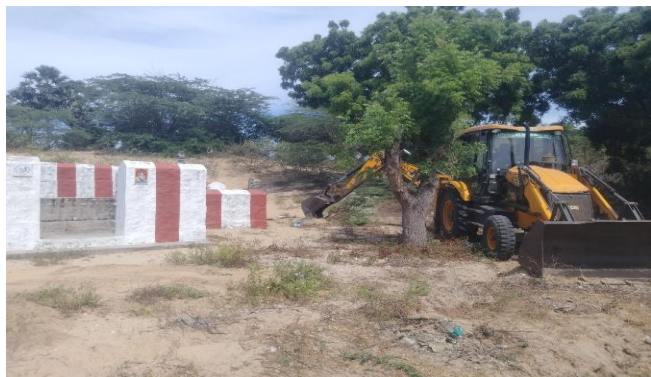
Cleaning work in progress at Krishna Teertham by using a JCB
